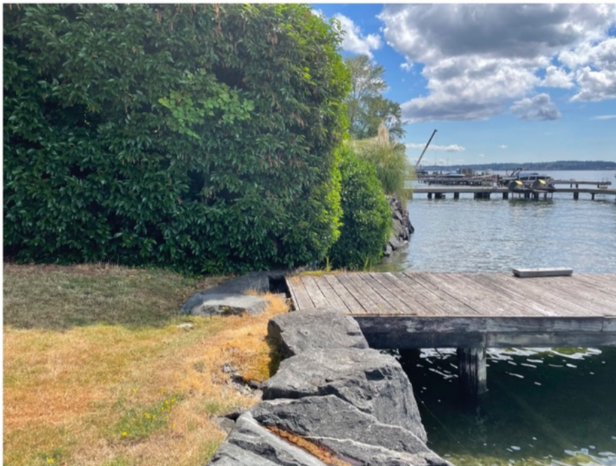
Photo 4 - Shoreline conditions looking south.
