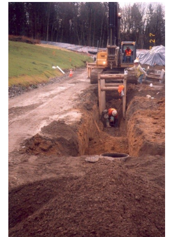
Gravity Sewer Line via Open Cut Construction
