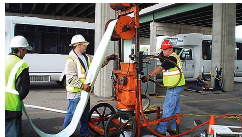
Cured-in-Place Pipe (CIPP)
