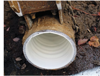
Gravity Sewer Line via Trenchless Technology
