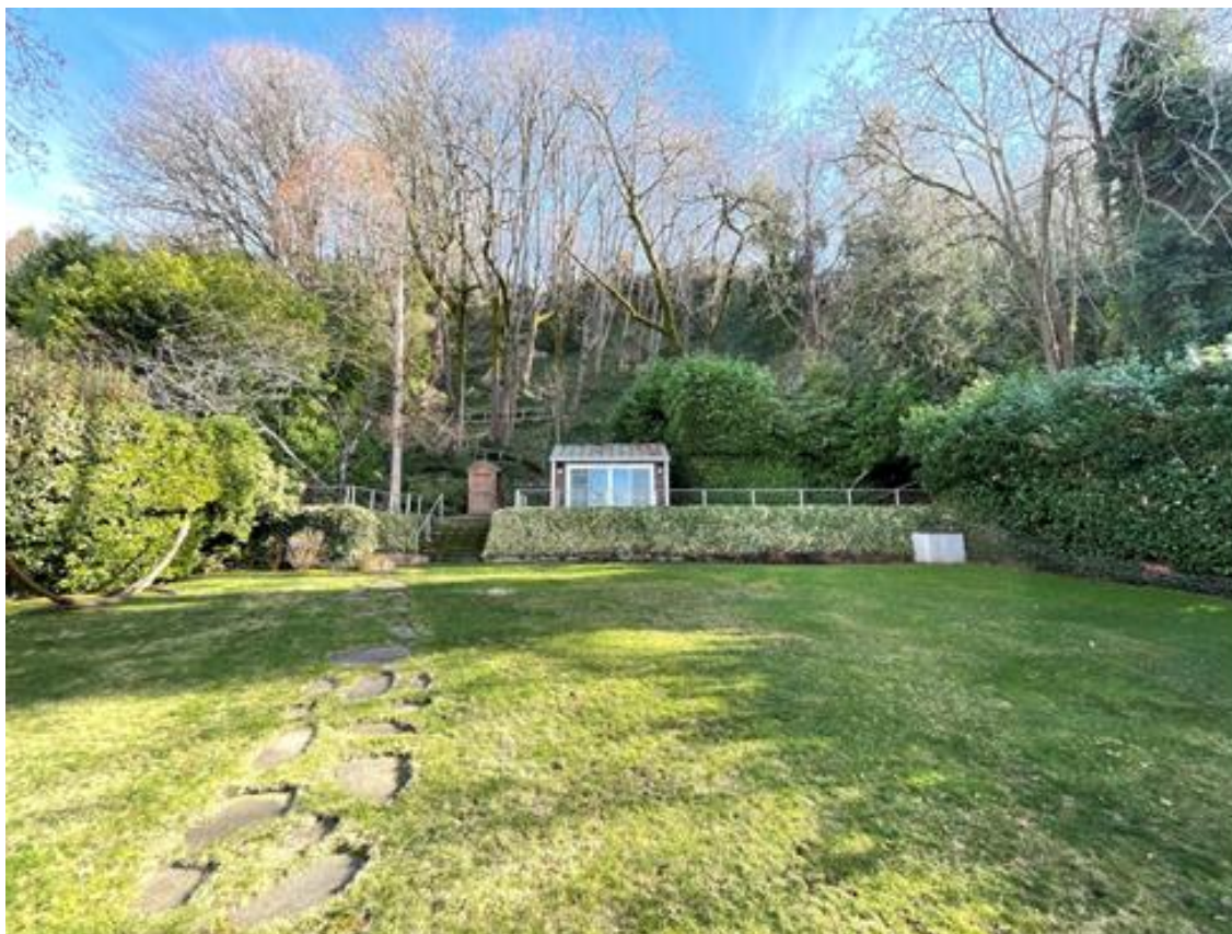
Plate 1. View of the existing shed, outbuilding and retaining wall along the toe of the slope. Looking east from Lake Washington shoreline
