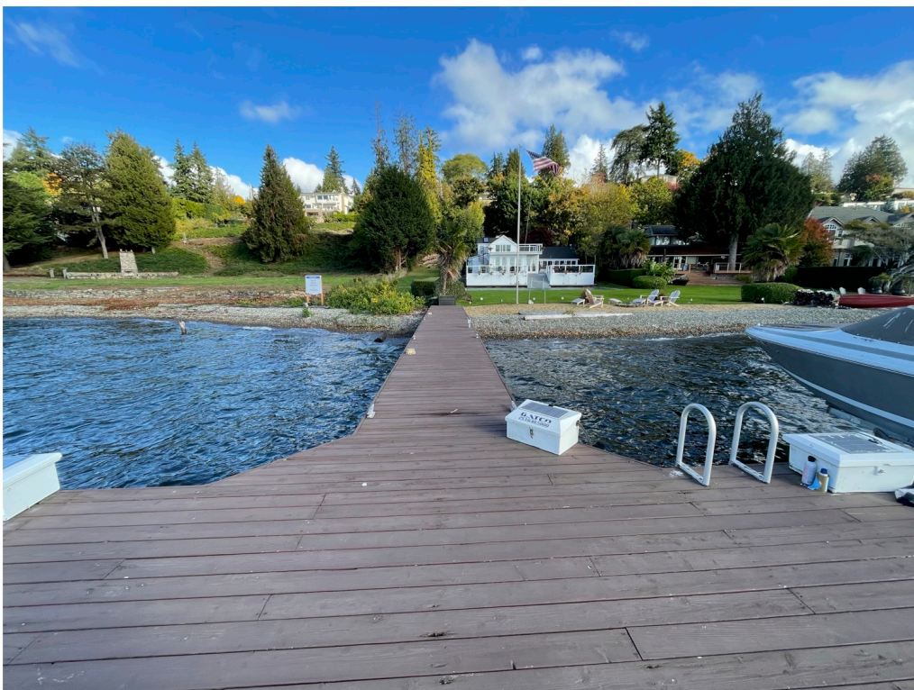
Photo 2 - Existing dock looking landward.
