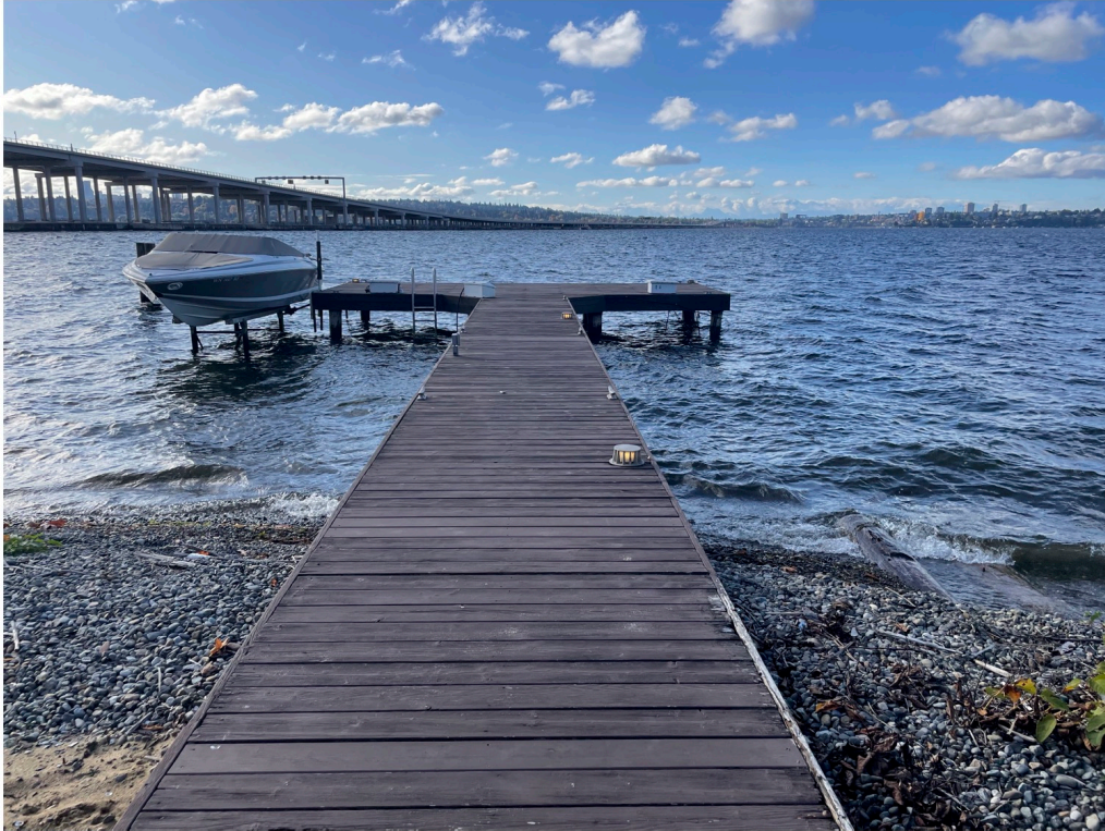
Photo 1 - Existing dock looking waterward.
