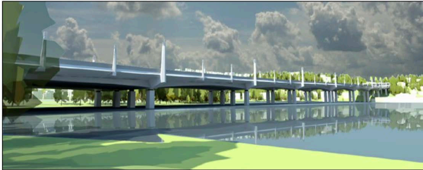
Rendering of a box girder conceptual design of Portage Bay Bridge, looking southwest. Final Concept Design Report, 2016.
