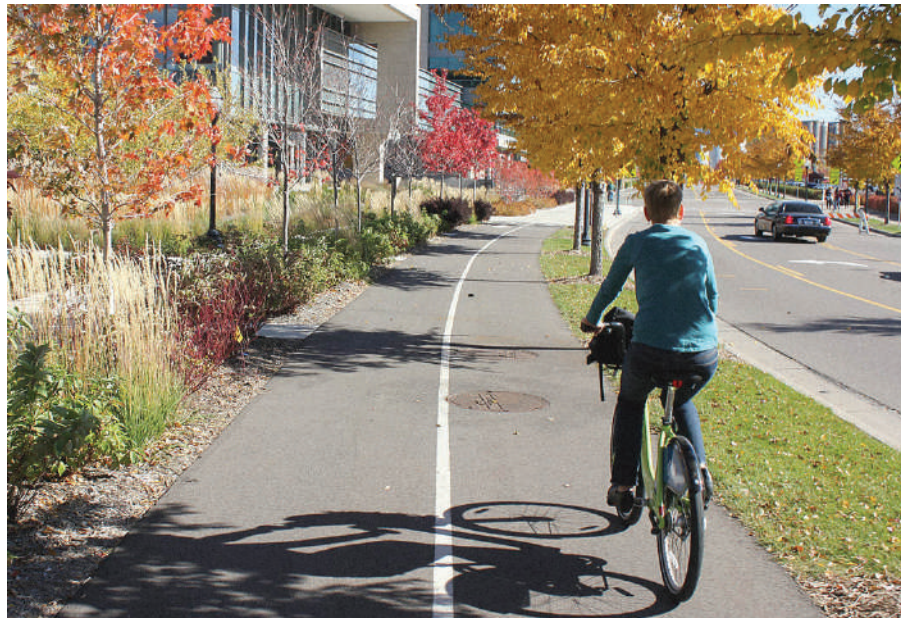
A shared use path is typically wider than a traditional sidewalk and is designed to accommodate pedestrians and cyclists.
