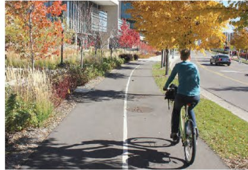
A shared use path is typically wider than a traditional sidewalk and is designed to accommodate pedestrians and cyclists.
