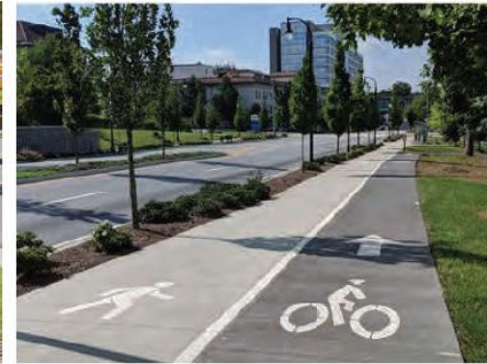
Lane markings and changes in material can be used to define various uses.
