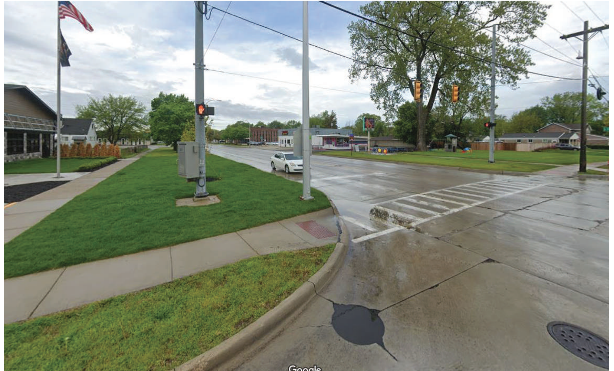
Existing Conditions on 11 Mile at Lorenz
