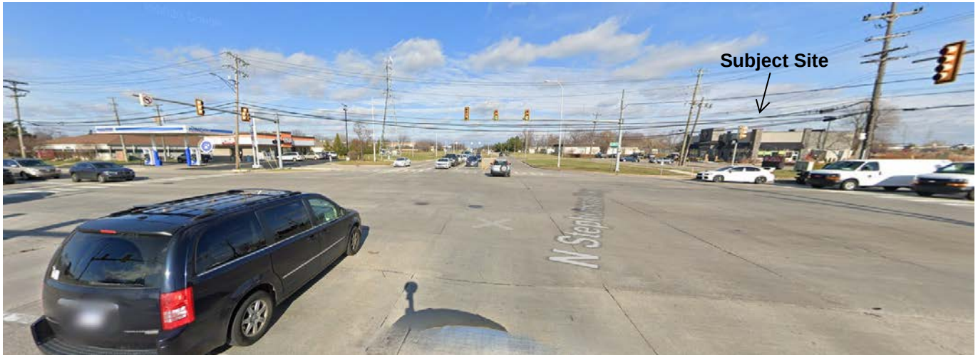
Existing Conditions at Stephenson/12 Mile (looking south)
