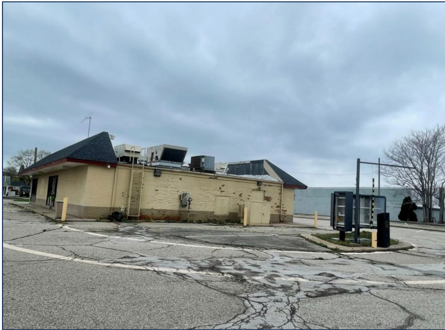
Exterior – Rear of Building
