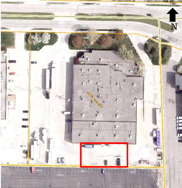
Existing Storage Conditions
