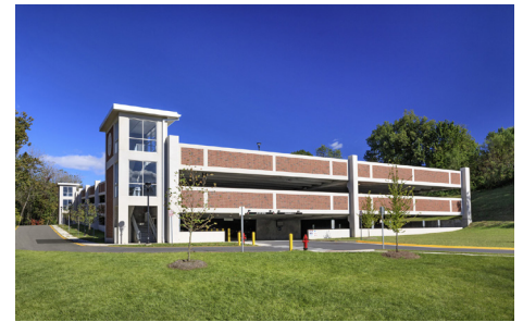
Shenandoah University Parking Garage I Winchester, VA
