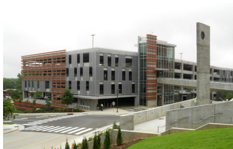
Wake Tech Health Sciences Building Parking Deck I Raleigh, NC
