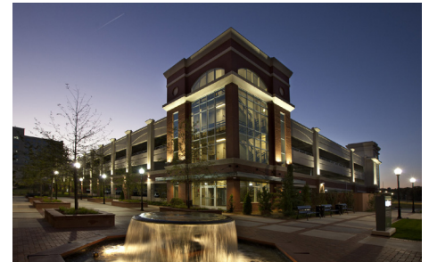
Saint John Street Parking Garage I Spartanburg, SC
