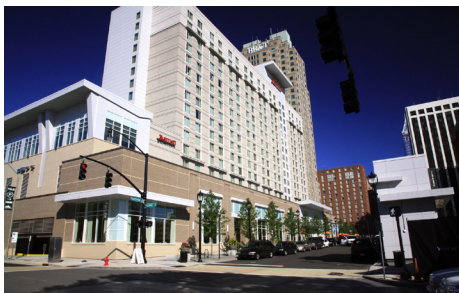
Downtown Underground Parking Facility | Raleigh, NC
