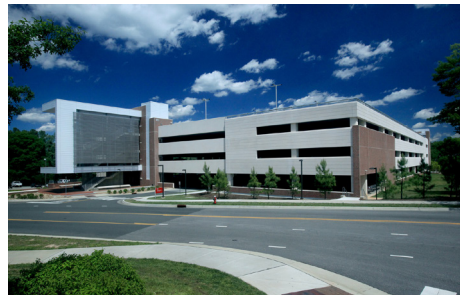
NC State University West Lot Parking Deck I Raleigh, NC
