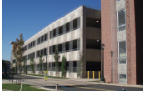
UVA Arts Ground Parking Garage I Charlottesville, VA
