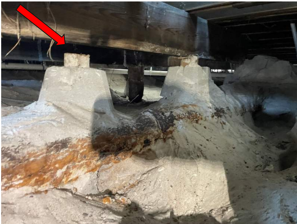
Photo 10 – Previous Retrofit with Detached Post
