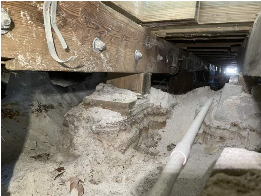
Photo 12 – Previous Retrofit of Sistered Beam
