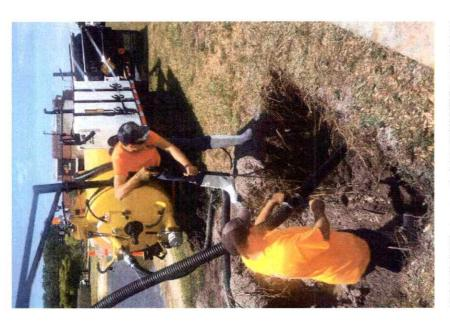
Above) An i2 Visual's team shown using their Hydro-Vac machine to dig close to utilities without damaging them. This is a very useful machine to avoid issues on today's crowed installation sites.
