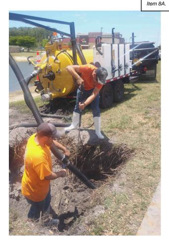
Above) An i2 Visual's team shown using their Hydro-Vac machine to dig close to utilities without damaging them. This is a very useful machine to avoid issues on today's crowed installation sites.
