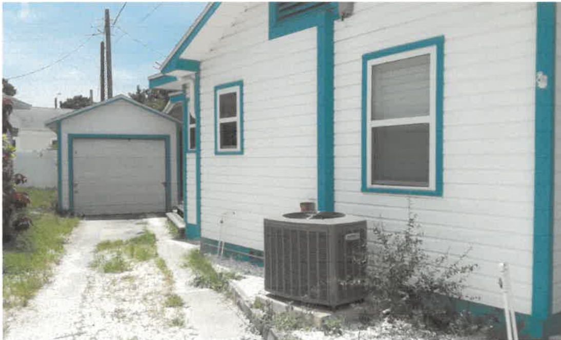
Photo Two Caption Photo Taken 07/31/2019 "Side View with A/C"
