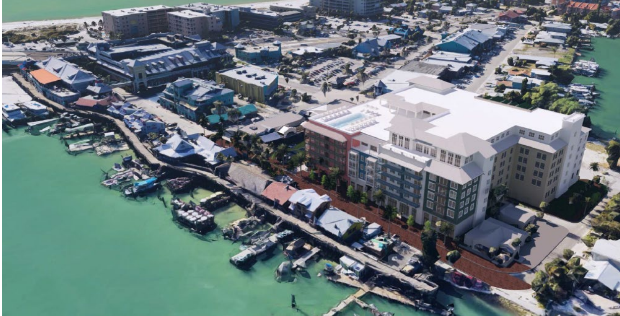
Closeup of the park showing the restroom building on the left and the small stage in the middle:
