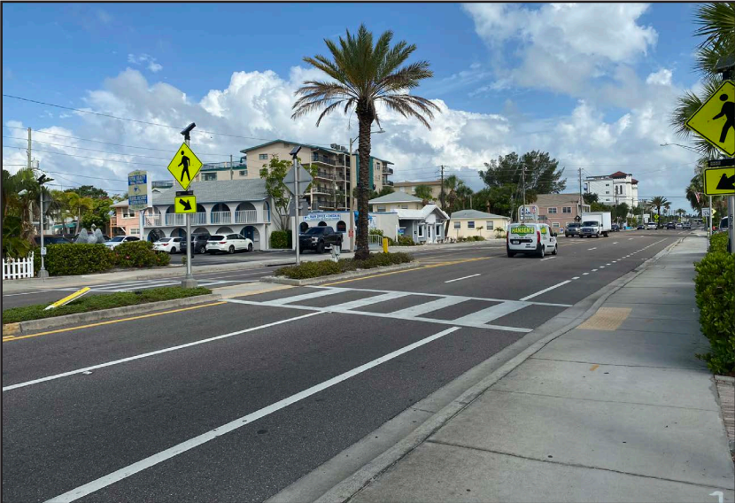
An example of landscaped median on Gulf Boulevard with bike lanes and a pedestrian crosswalk.
