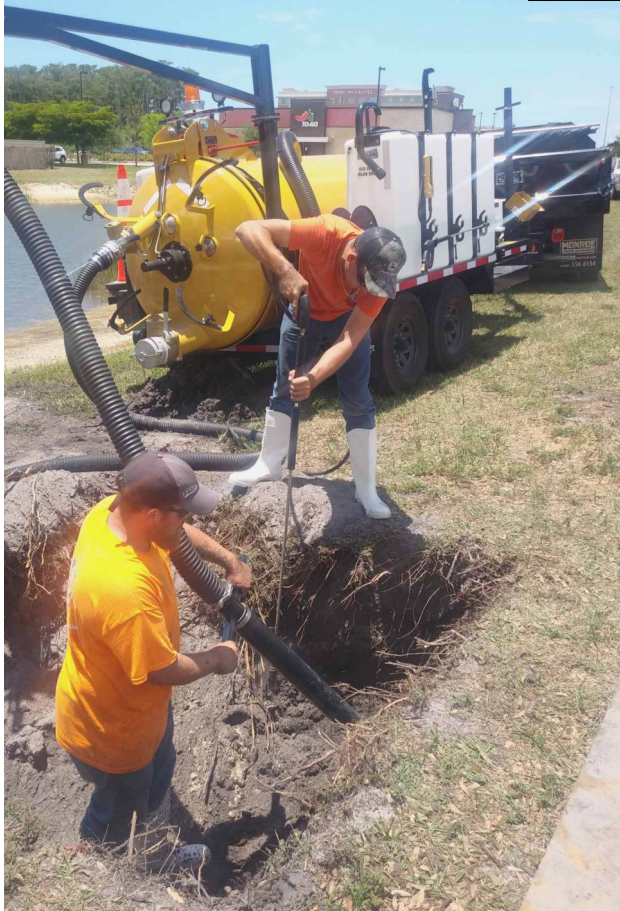
Above) An i2 Visual's team shown using their Hydro-Vac machine to dig close to utilities without damaging them. This is a very useful machine to avoid issues on today's crowded installation sites.
