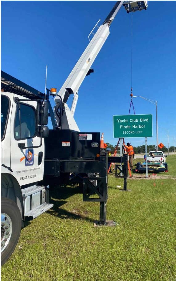
Above) One of i2 Visual's experienced install teams finishing one of two new FDOT standard multi-post traffic signs for Charlotte County Florida (footers, break-away structure and sign panel.)
