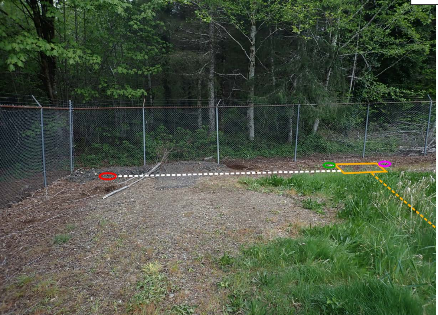
Image 5: Looking north at the station configuration for 1207-DOORS. The post-hole sensor (marked by red circle) will be located in the northwest corner of the fenced-in utility compound. The post and power enclosure (marked by the orange rectangle) will be located approximately 20 ft to the east of the post-hole sensor, along the north fence line of the utility compound. Cabling (dashed white lines) between the sensor and the post and power enclosure will be trenched. Power for the instrument will be provided by an outdoor pole-mounted 120v AC connection located approximately 16m to the southeast. AC power will be converted to low-voltage DC current and trenched to the post and power enclosure (orange dashed line). The trench path for the low-voltage power cable will depend on the location of buried utilities (fiber). A GPS antenna (green circle) will be mounted to the post and power enclosure. A Nanobeam puck (purple circle) will be mounted to the post and power enclosure and pointed to the comms shack in the northeast corner of the fenced-in utility compound where contractors will mount a second Nanobeam puck.
