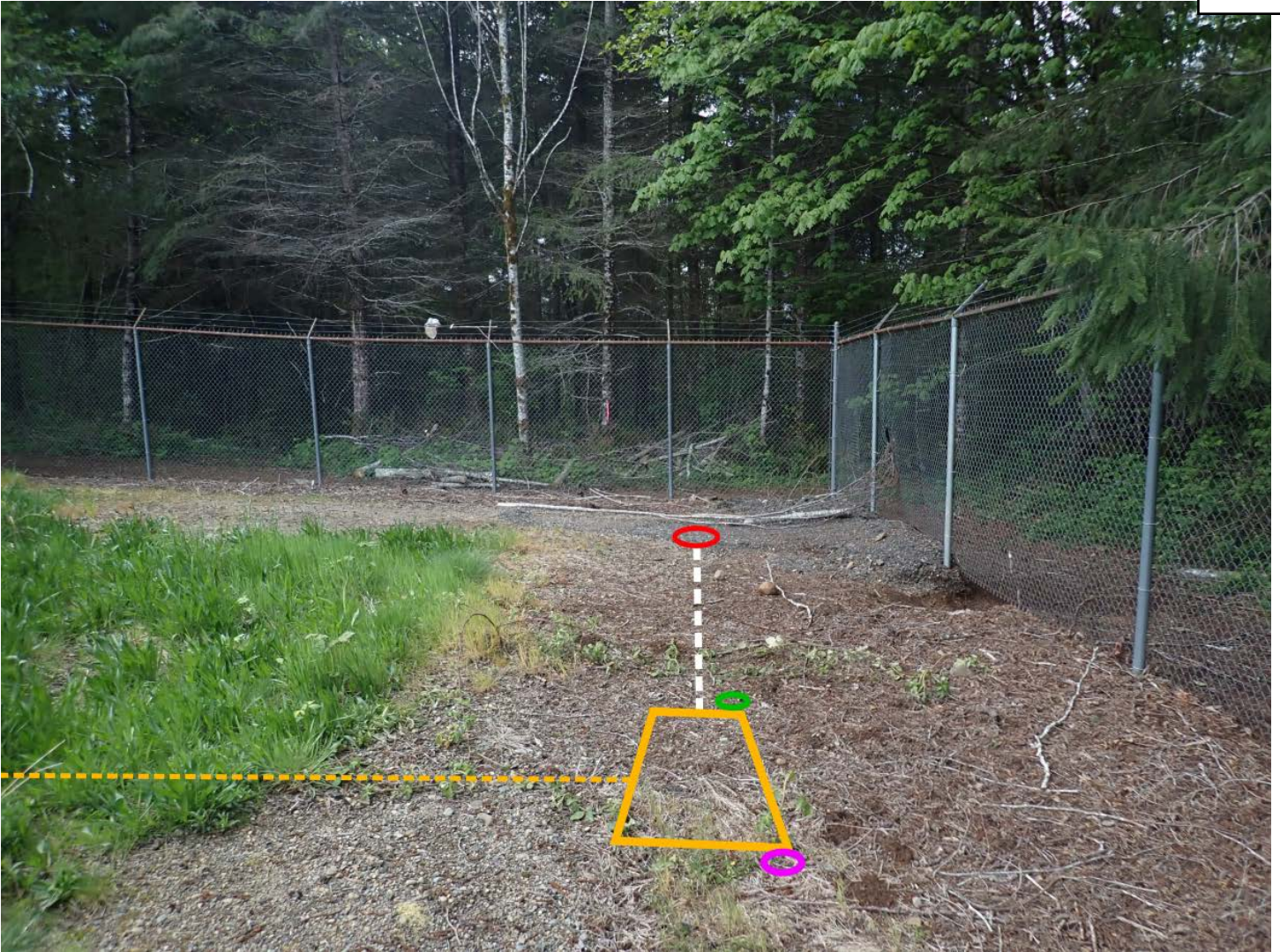
Image 6: Looking west at the station configuration for 1207-DOORS. The post-hole sensor (marked by red circle) will be located in the northwest corner of the fenced-in utility compound. The post and power enclosure (marked by the orange rectangle) will be located approximately 20 ft to the east of the post-hole sensor, along the north fence line of the utility compound. Cabling (dashed white lines) between the sensor and the post and power enclosure will be trenched. Power for the instrument will be provided by an outdoor pole-mounted 120v AC connection located approximately 16m to the southeast. AC power will be converted to low-voltage DC current and trenched to the post and power enclosure (orange dashed line). The trench path for the low-voltage power cable will depend on the location of buried utilities (fiber). A GPS antenna (green circle) will be mounted to the post and power enclosure. A Nanobeam puck (purple circle) will be mounted to the post and power enclosure and pointed to the comms shack in the northeast corner of the fenced-in utility compound where contractors will mount a second Nanobeam puck.
