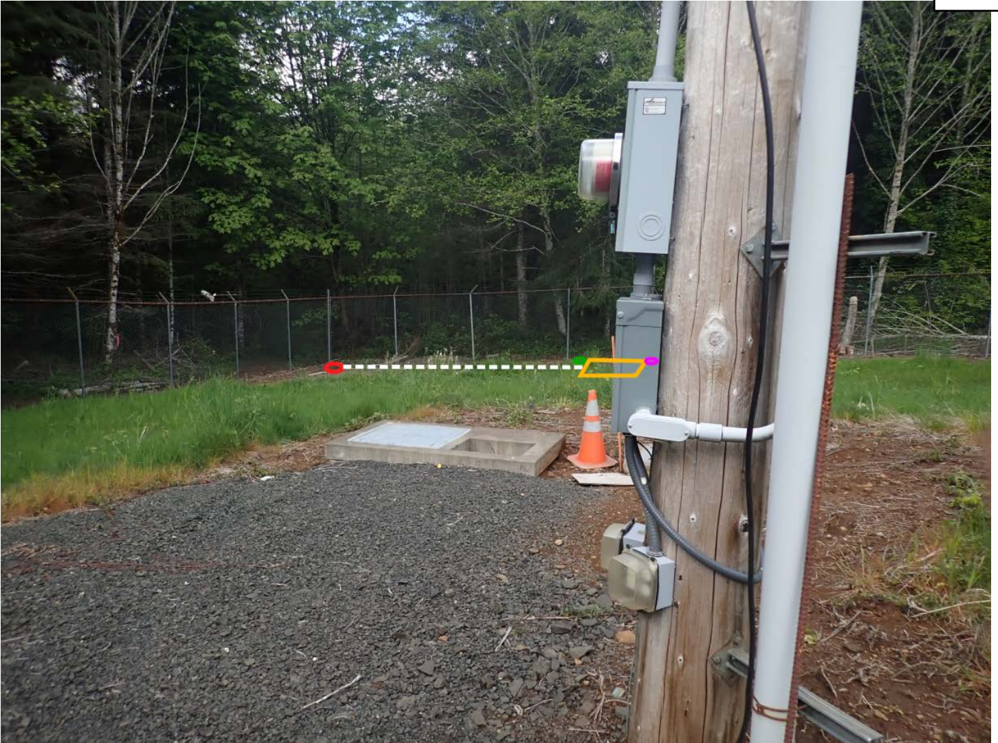
Image 8: Looking north northwest at the AC power pole that will provide power for the instrument. The proposed station location is depicted in the background of the image. AC power will be converted to low voltage DC power and trenched to the post and power enclosure. The precise path of trenching will depend on the location of other buried utilities (fiber). A small repeater box will need to be mounted to the power pole to host the AC to DC power converter. An electrician will need to be onsite to pull power from the power pole.
