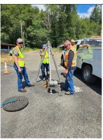
the gas sniffer to detect any unsafe gases before entering the manhole.
