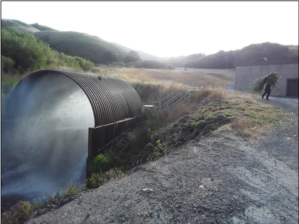
Photo 20: Facility Maintenance at the Soulajule Dam
