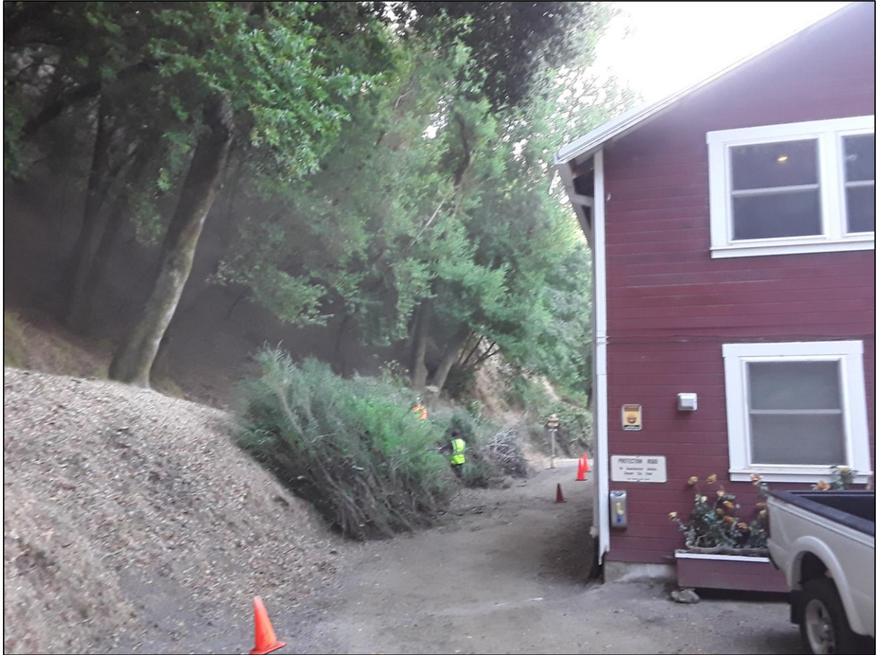
Photo 21: MWPA Contractors building Fuelbreak adjacent to Marin Stables.
