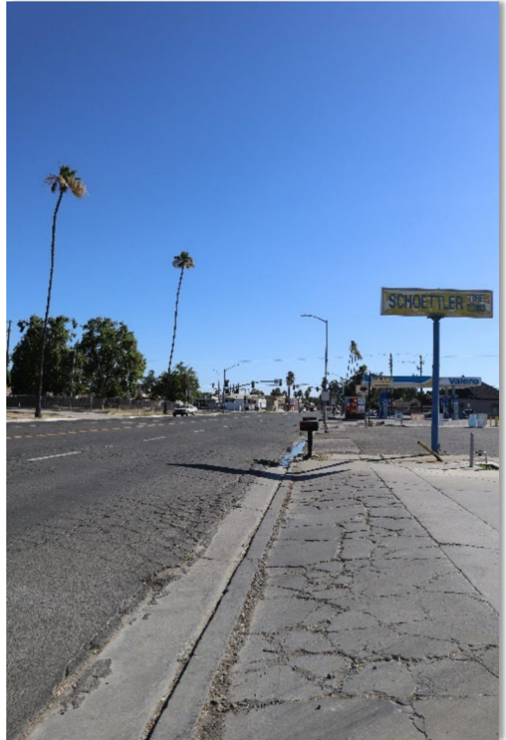
Figure 11: SR 233 between Washington Rd and 15th St - cracks in driveway and pavement
