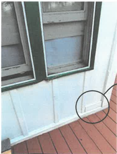
Patched rot holes in exterior wall
