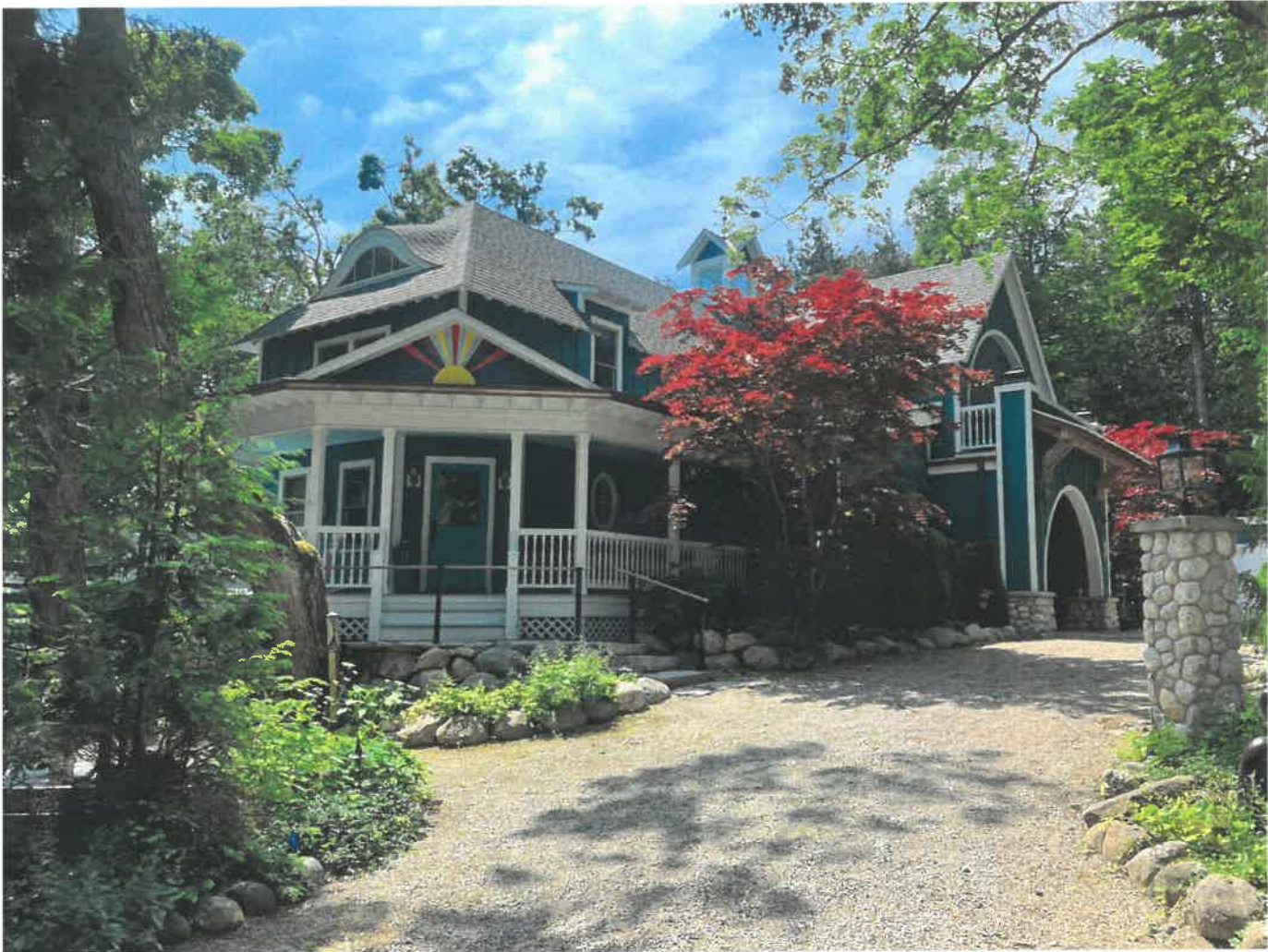
Adjacent carriage house, 8200 Lakeview Blvd, from Grand Ave. looking West
