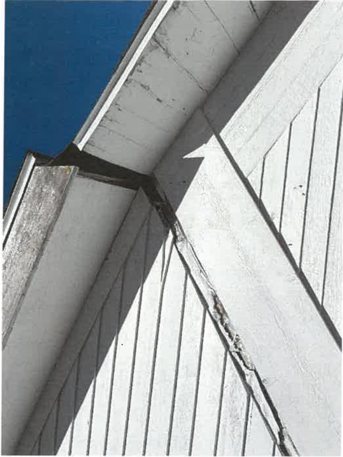
Back of Parapet
