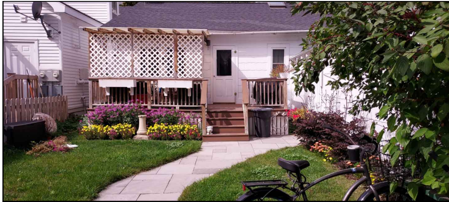
ALLEY VIEW OF EXISTING ROSE UNIT
