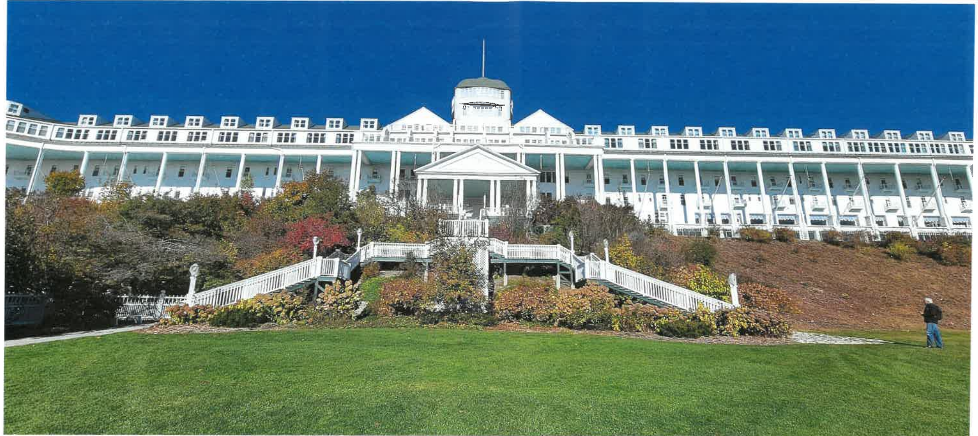
STAIRS LOOKING NORTH
