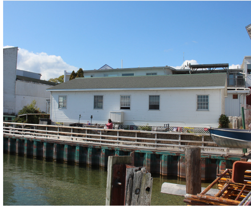
EXISTING SHED AND SEA WALL, LOOKING NORTH
