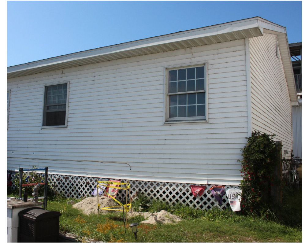
CORNER OF EXISTING SHED, LOOKING NORTHWEST
