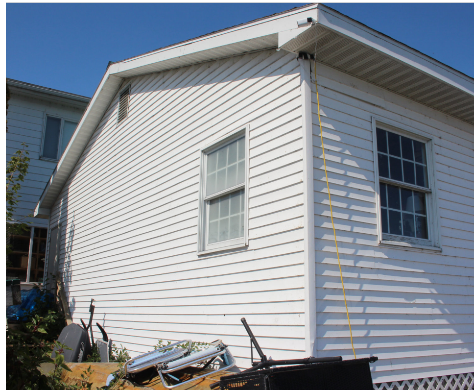
CORNER OF EXISTING SHED, LOOKING NORTHEAST
