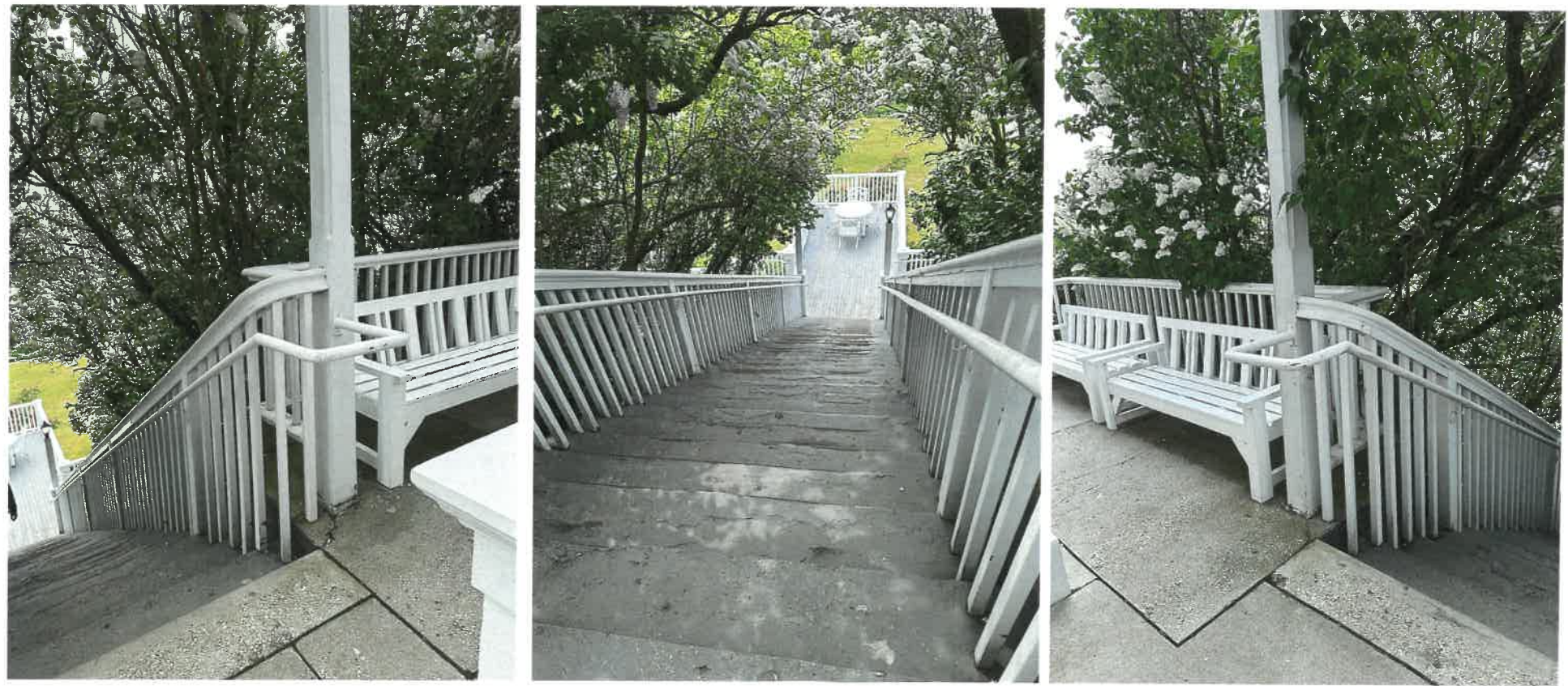
TOP OF STAIRS LOOKING SOUTH
