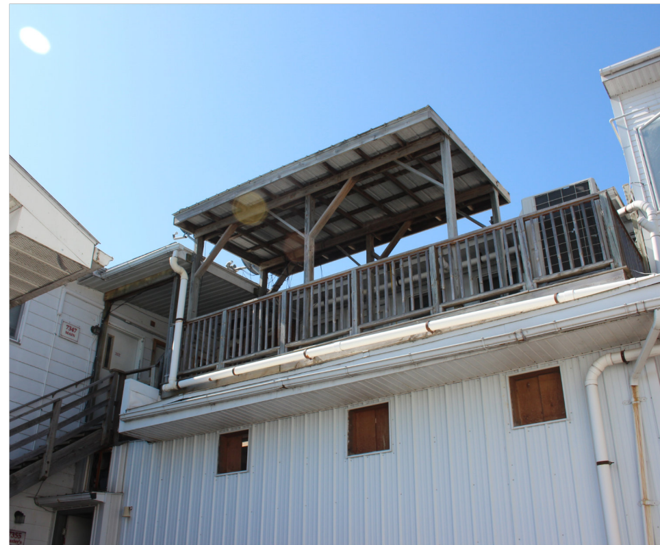
EXISTING UPPER PORCH AND EXISTING SOUTH EXTERIOR WALL, LOOKING NORTH
