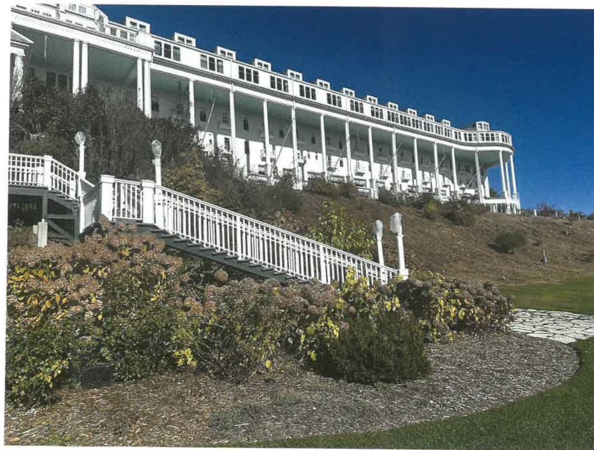
LOWER WEST STAIR
