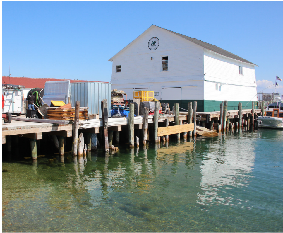
NEIGHBORING BUILDING, LOOKING SOUTHEAST FROM DECK
