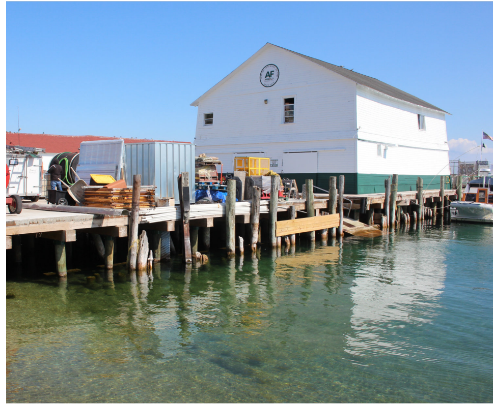
NEIGHBORING BUILDING, LOOKING SOUTHEAST FROM DECK
