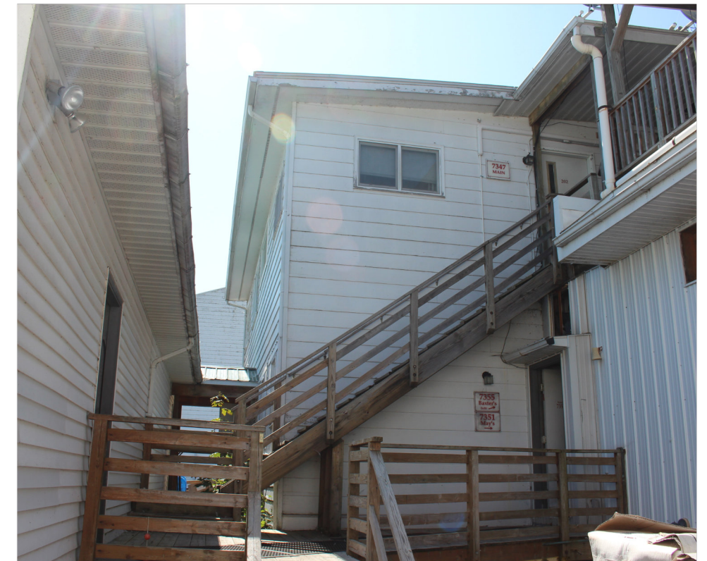
EXISTING WOODEN STRUCTURE, PORCH AND STAIR CONNECTING EXISTING SHED AND BUILDING, LOOKING WEST
