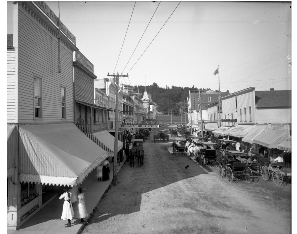
MACKINAC ISLAND MAIN STREET LOOKING NORTH FROM ASTOR STREET
