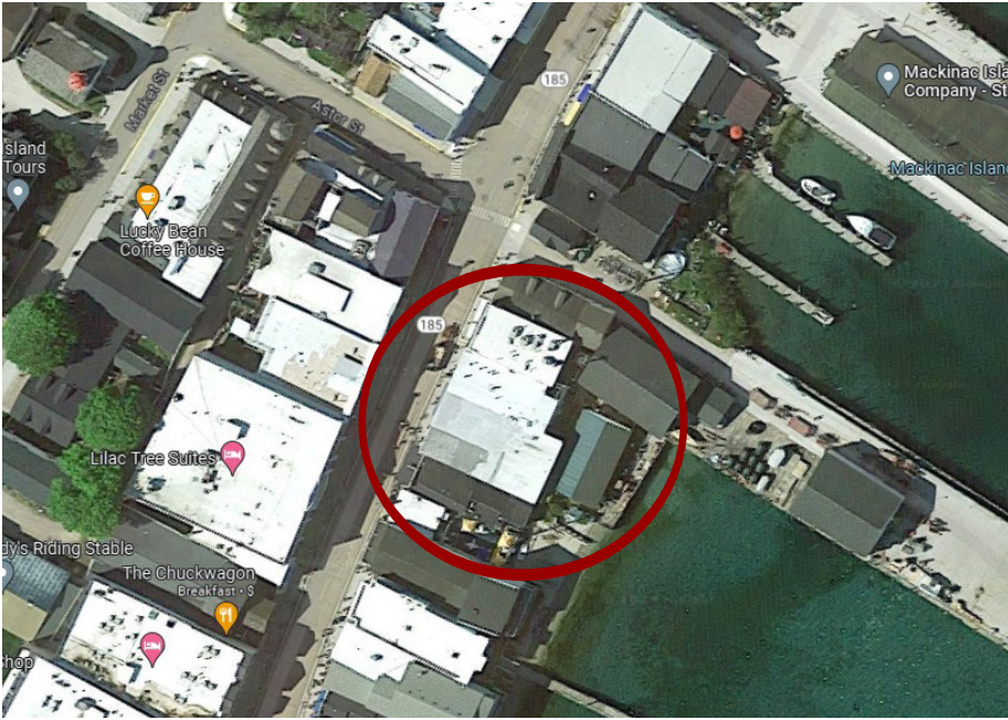
Figure 1-1. Aerial view of the subject building within the red circle (Google Maps, 2023).
