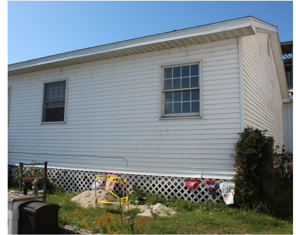
CORNER OF EXISTING SHED, LOOKING NORTHWEST
