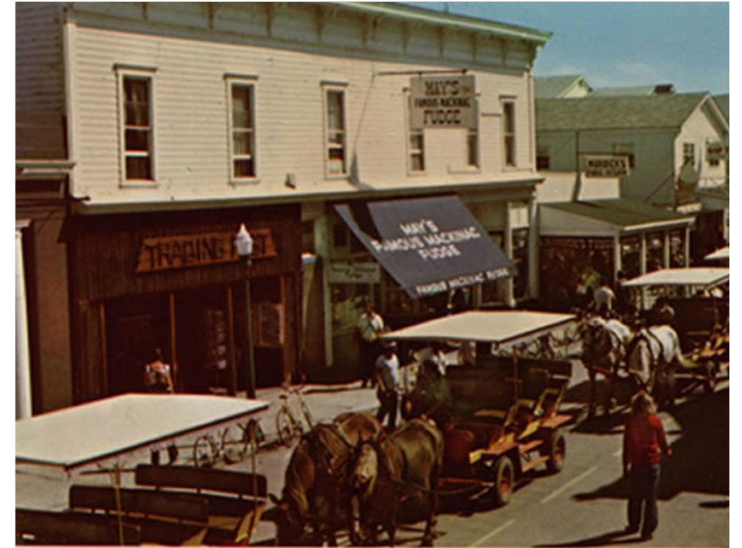
PROJECT BUILDING (date unknown)
