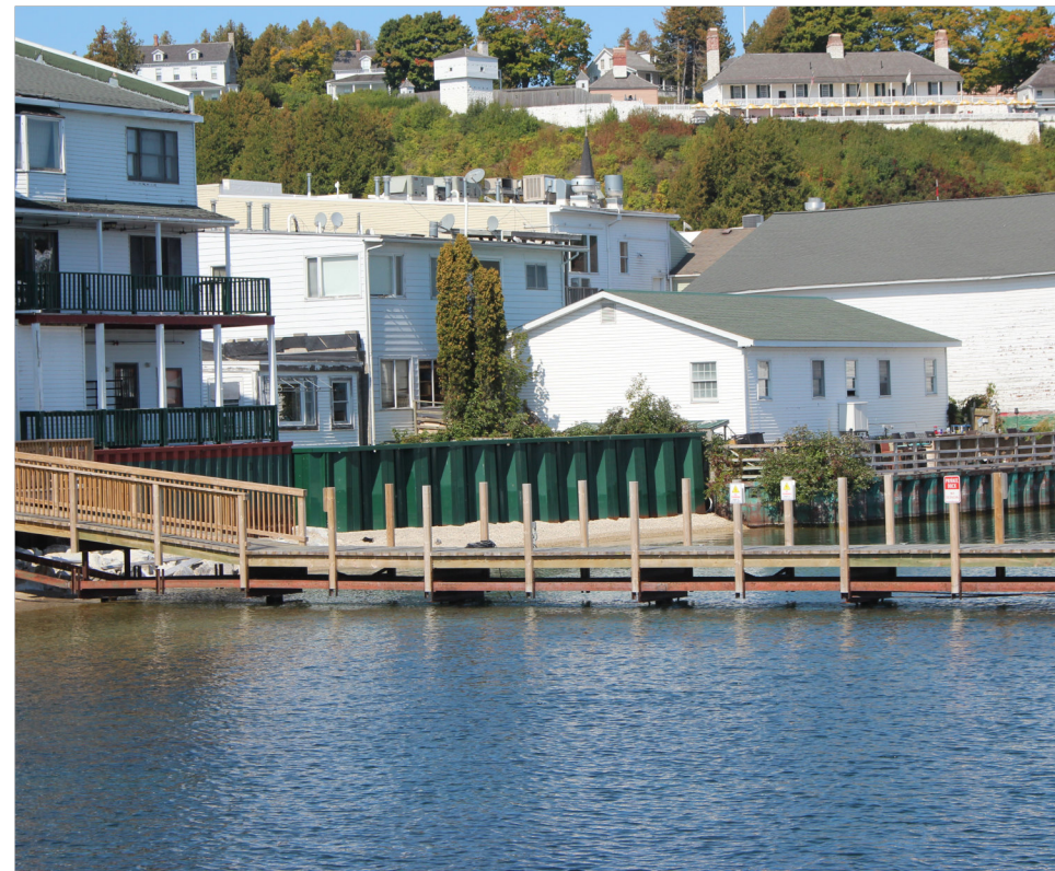
EXISTING BUILDING, SHED AND SEAWALL, LOOKING NORTHEAST
