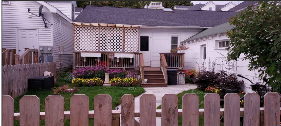
ALLEY VIEW OF EXISTING ROSE UNIT
