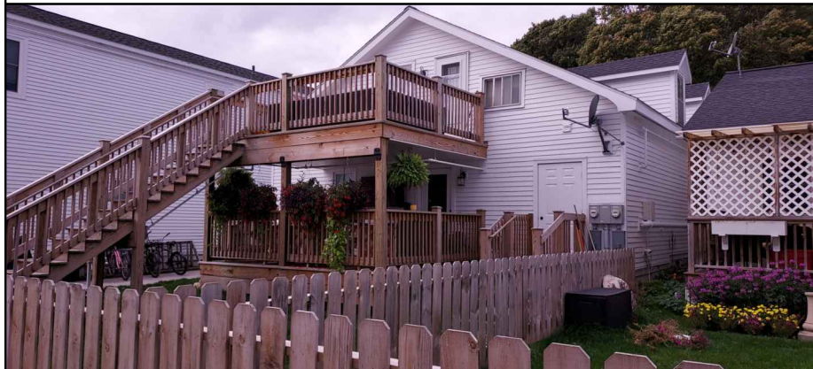
ALLEY VIEW OF GULL
