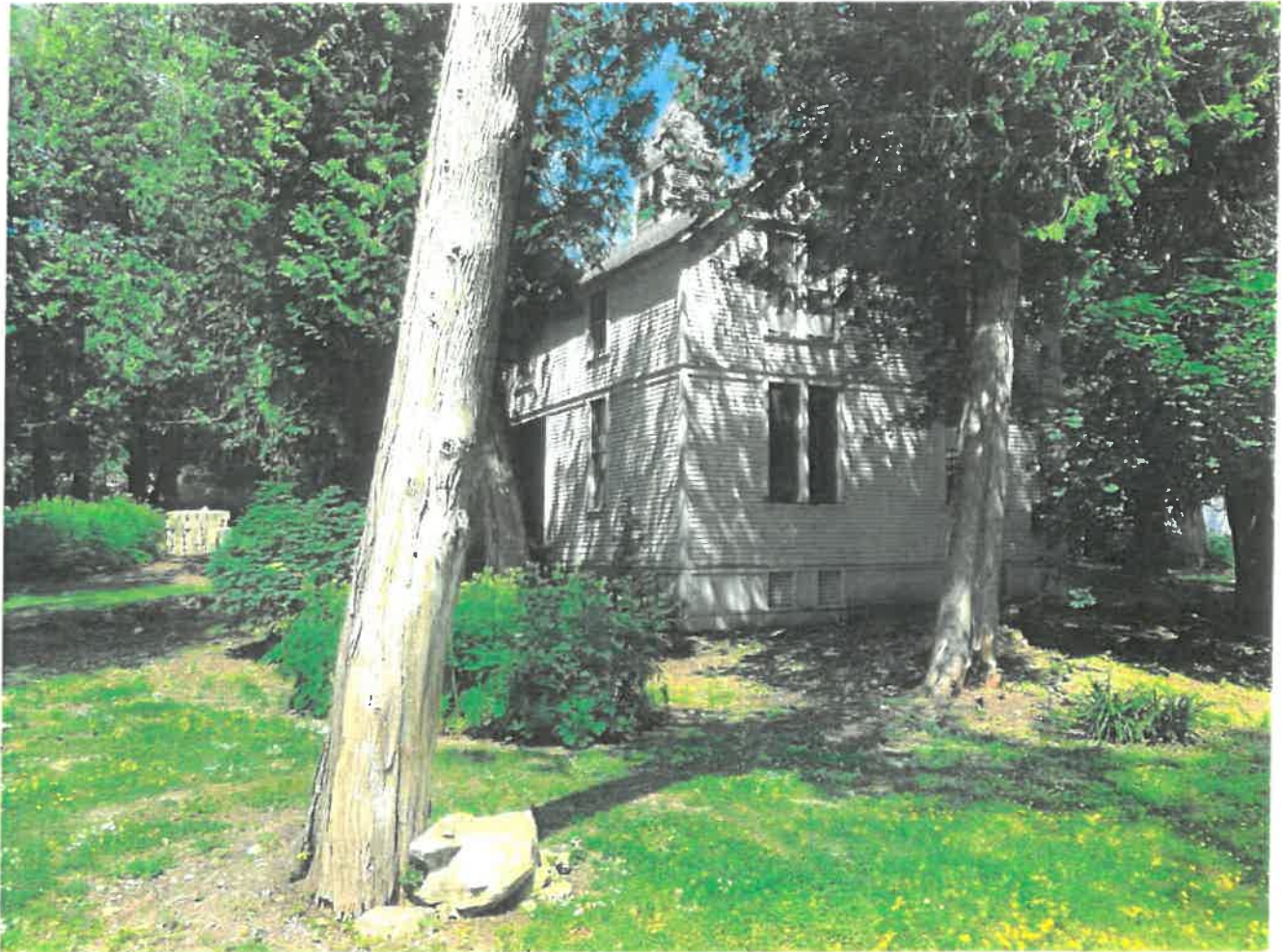
Adjacent carriage house, 8247 Lakeview Blvd, from Grand Ave, looking North
