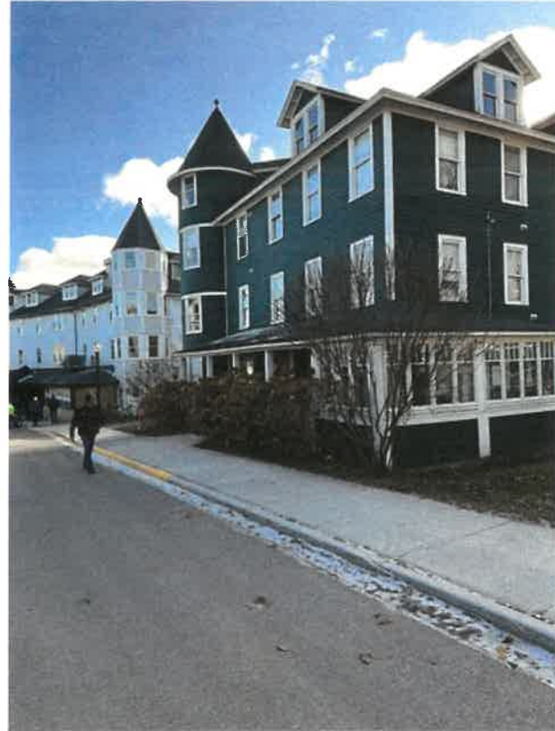
STREET FRONT OF BUILDING, LOOKING SOUTH
