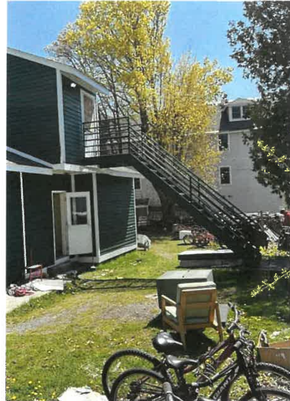
REAR EGRESS STAIR, LOOKING EAST
