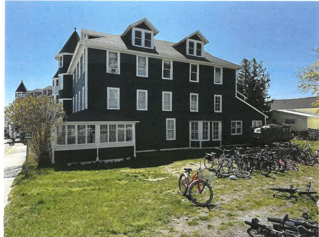
SIDE VIEW OF BUILDING, LOOKING SOUTH-EAST
