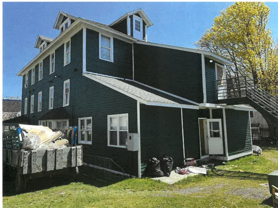
REAR OF BUILDING, LOOKING EAST
