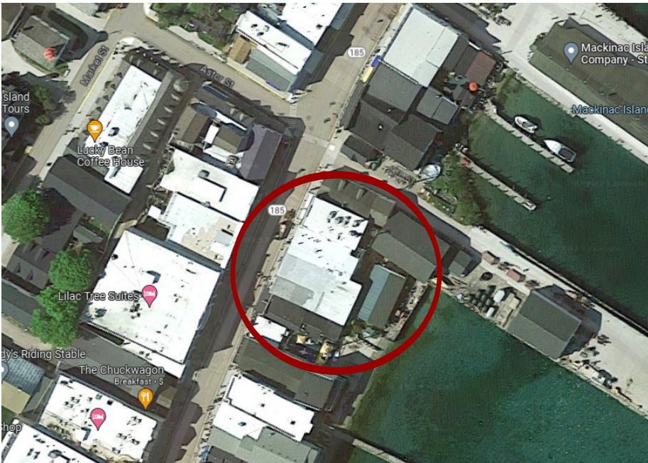
Figure 1-1. Aerial view of the subject building within the red circle (Google Maps, 2023).
