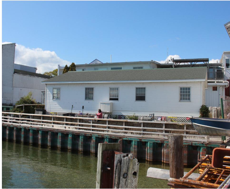
EXISTING SHED AND SEA WALL, LOOKING NORTH
