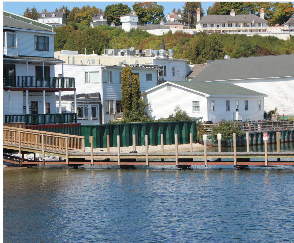
EXISTING BUILDING, SHED AND SEAWALL, LOOKING NORTHEAST
