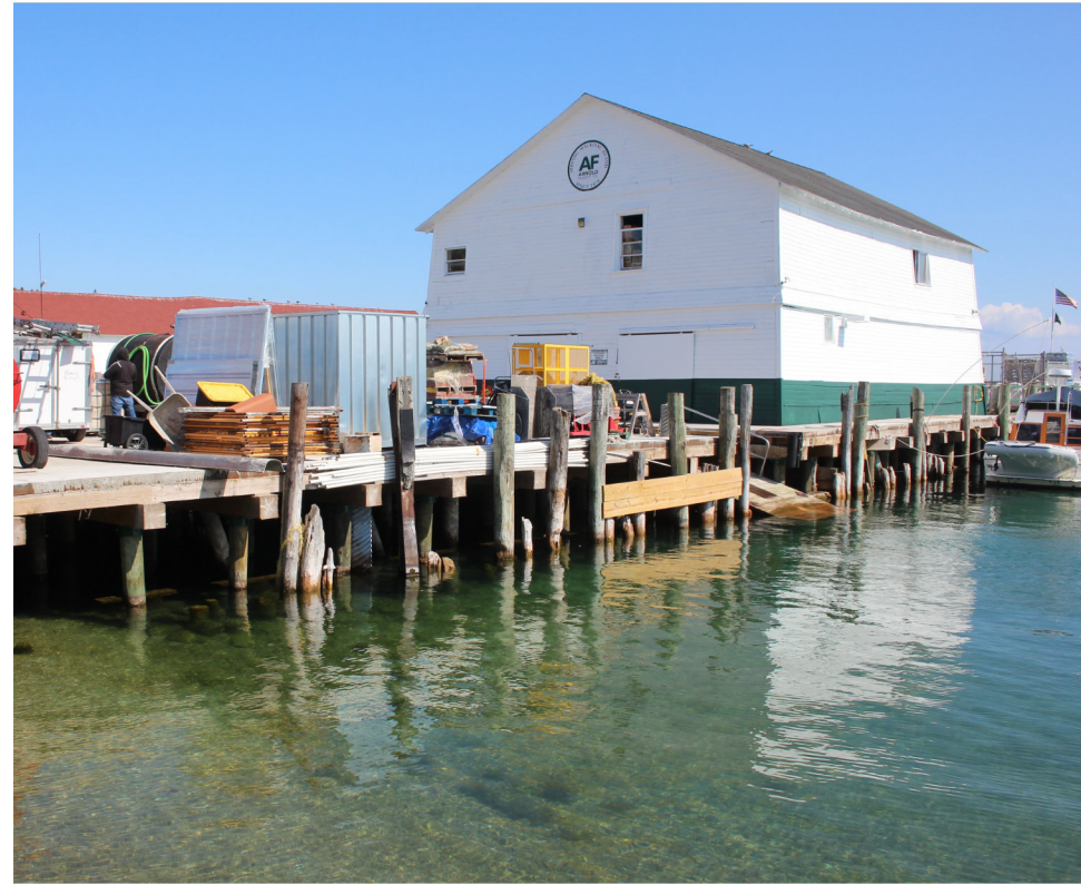
NEIGHBORING BUILDING, LOOKING SOUTHEAST FROM DECK
