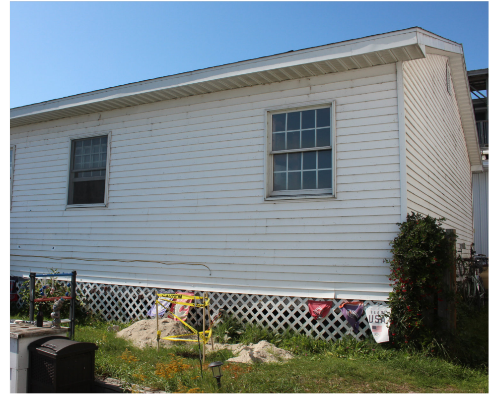
CORNER OF EXISTING SHED, LOOKING NORTHWEST
