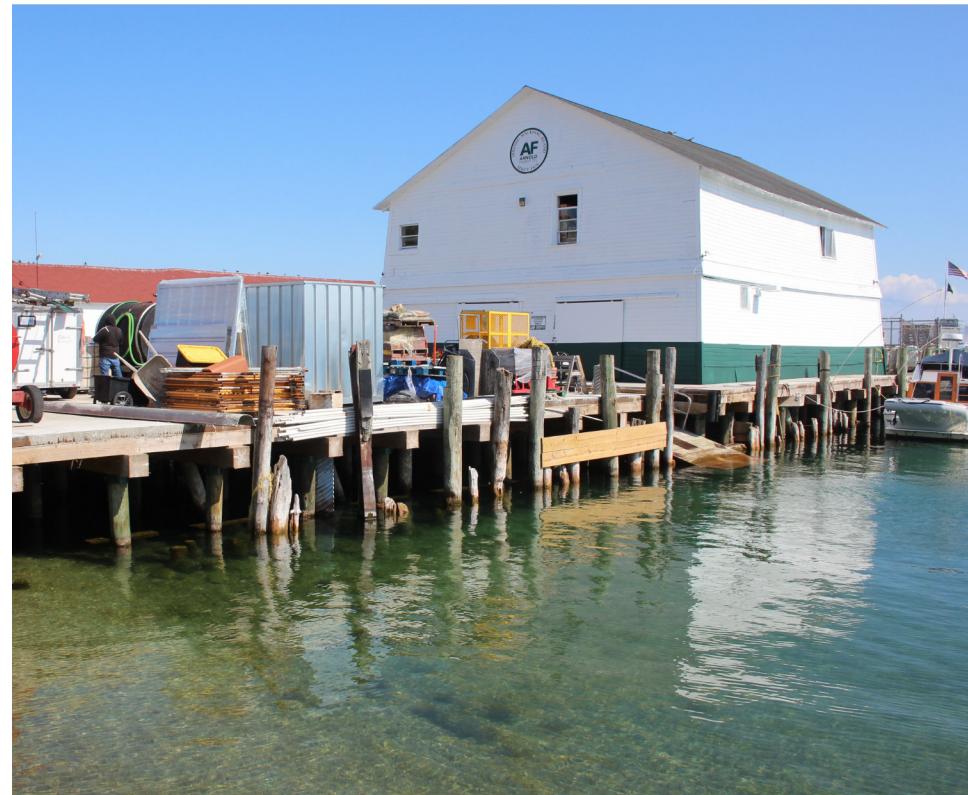
NEIGHBORING BUILDING, LOOKING SOUTHEAST FROM DECK
