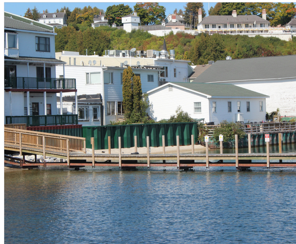
EXISTING BUILDING, SHED AND SEAWALL, LOOKING NORTHEAST
