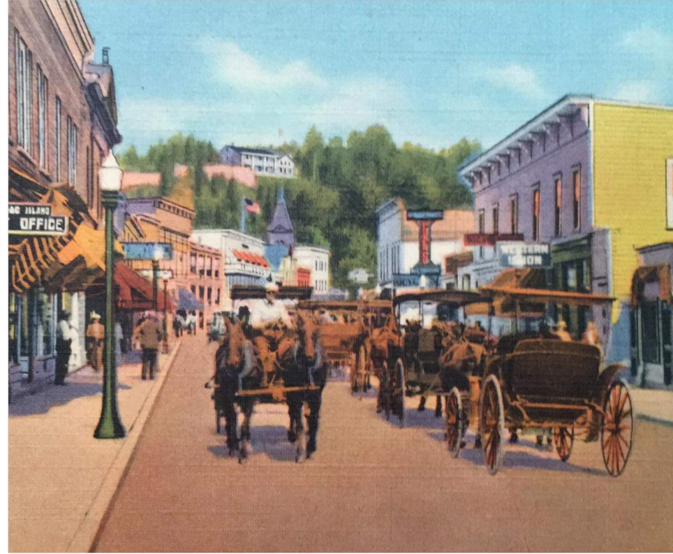
MACKINAC POST CARD - PROJECT BUILDING ON RIGHT SIDE
