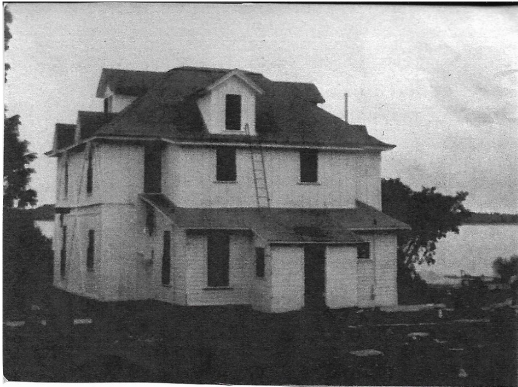
Rear elevation of cottage.
