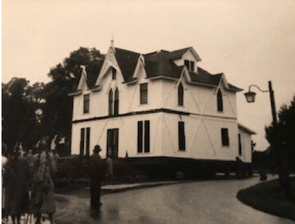
Cottage in process of move.
