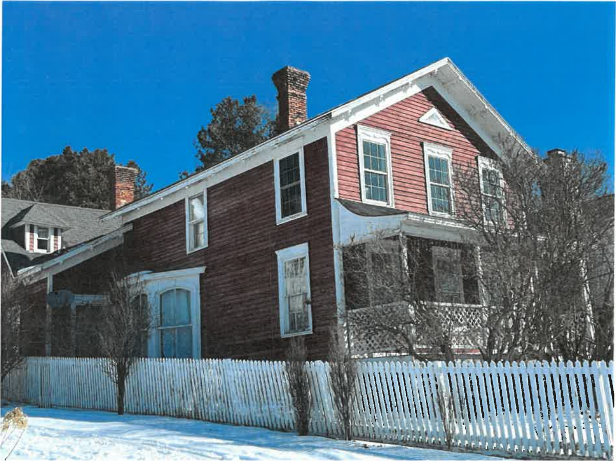
Photo 2. 6948 Main Street, c. 1850.
