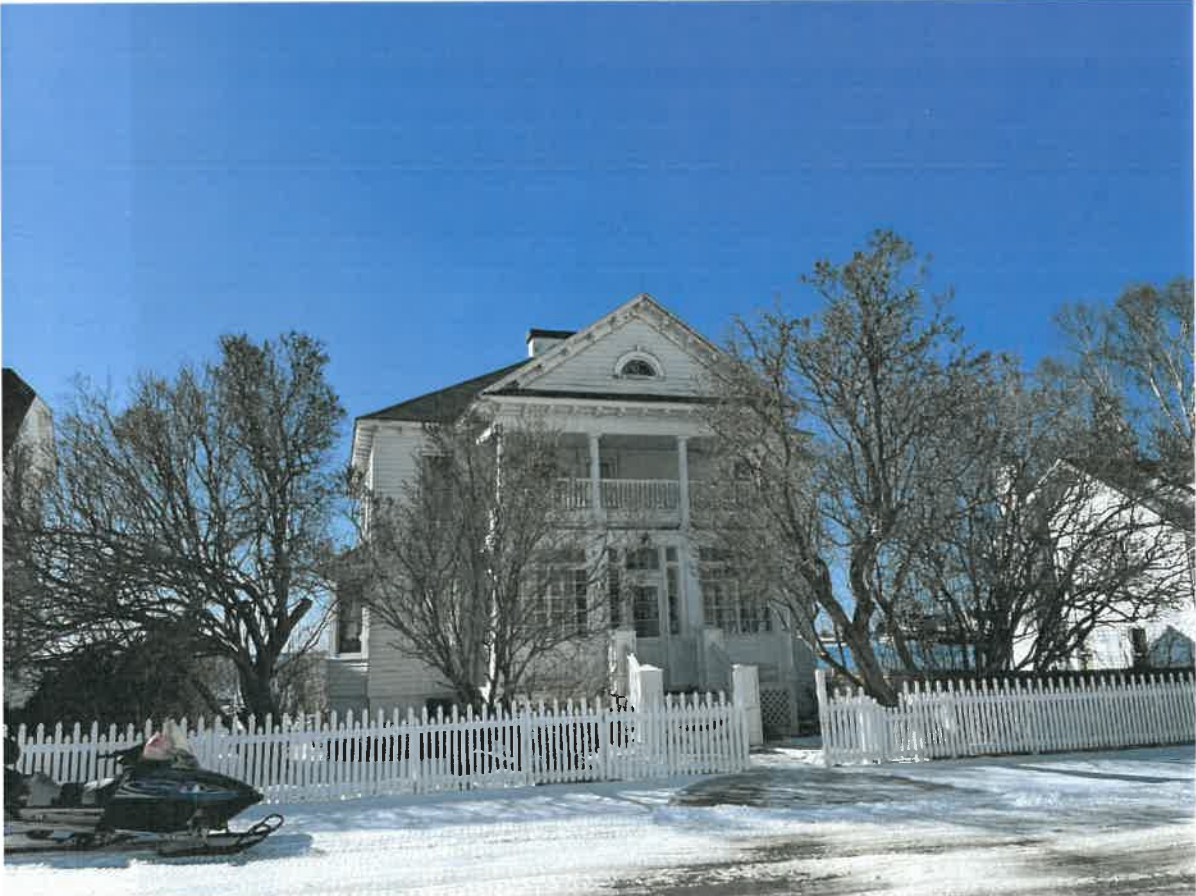
Photo 5. Saint Anne's Rectory, 6837 Main Street
