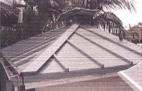
Standing Seam Sheet Metal
