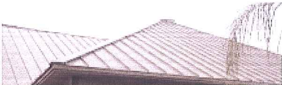
Standing Seam Sheet Metal
