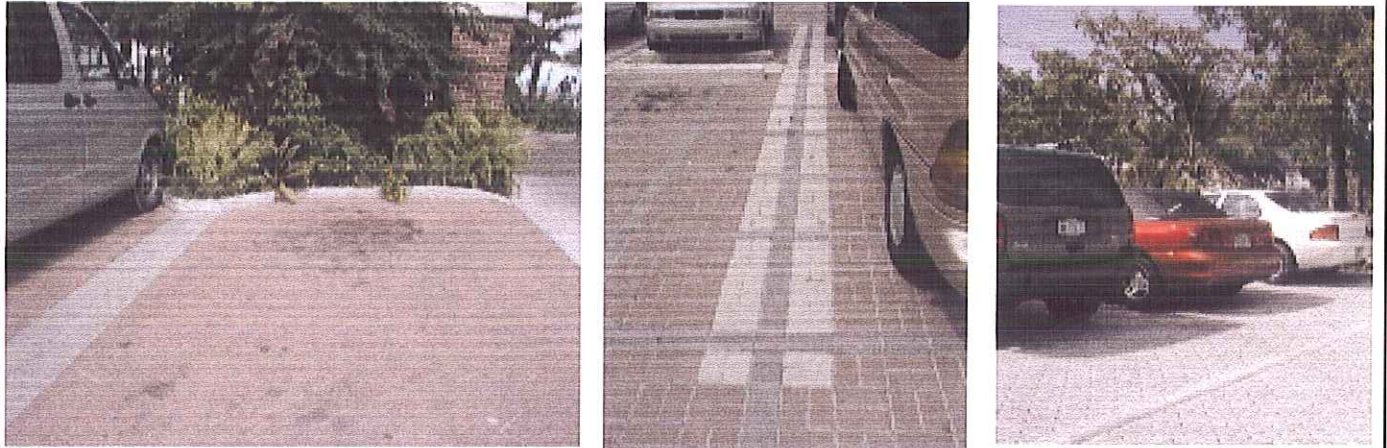
Colored Pavers to Mark Parking Places
