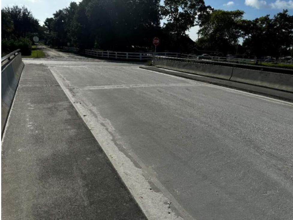
Photo 43 – View of concrete bridge running surface condition.
