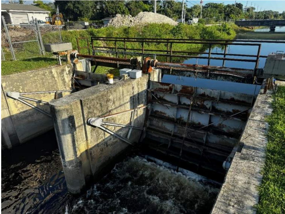
Photo 53 – View of radial flood gates, concrete wall and metal walkway at Control Structure D.
