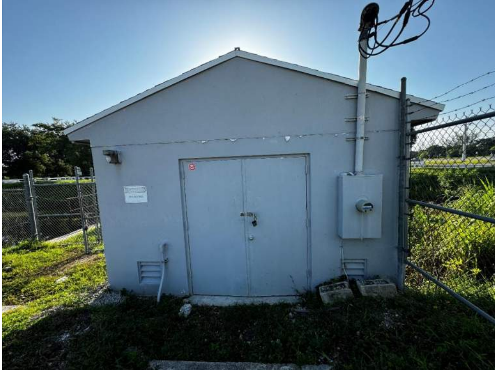
Photo 45 – View of floor pump-house west elevation.
