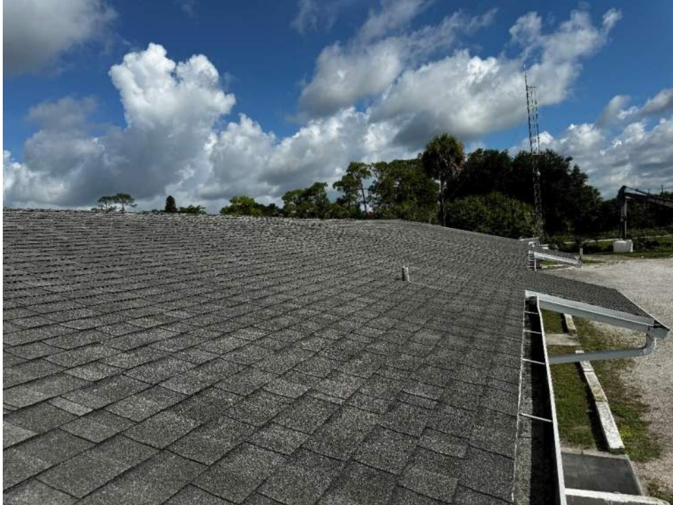
Photo 9 – View of office building roofing condition.
