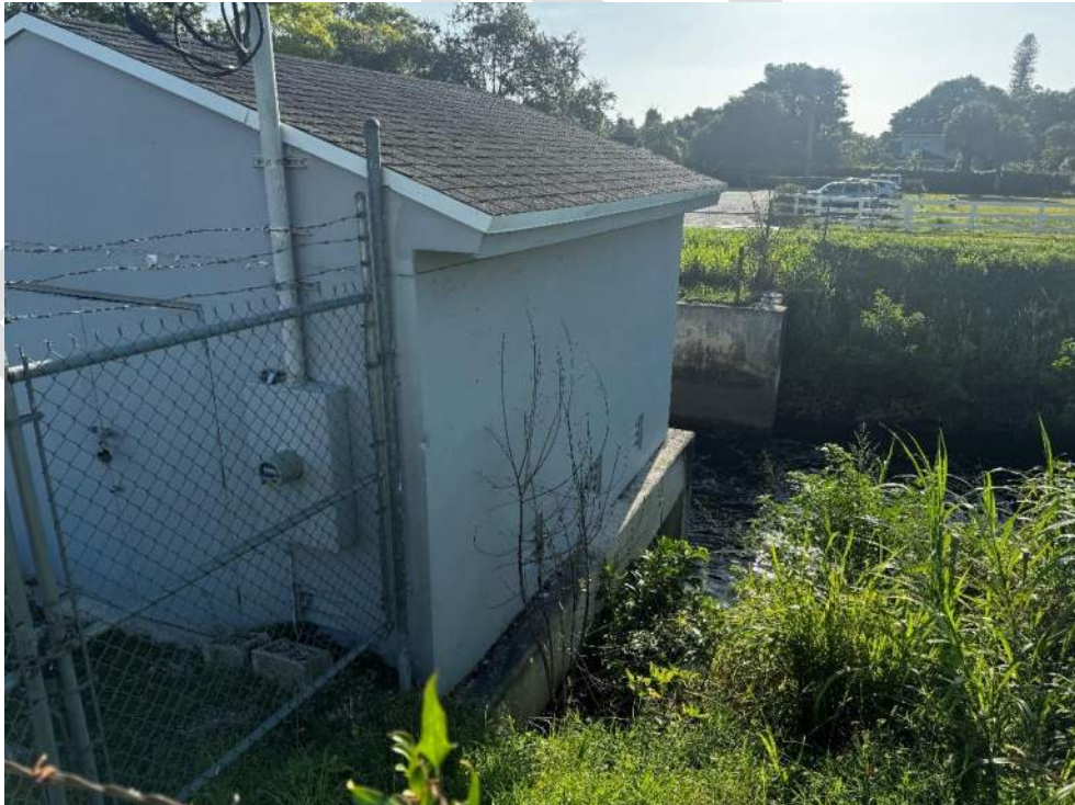
Photo 46 – View of floor pump-house southwest elevation.
