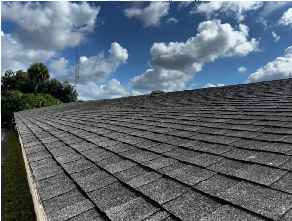
Photo 10 – View of office building roofing condition.
