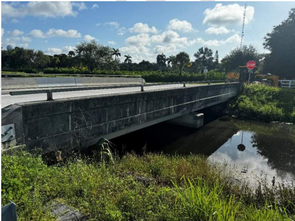
Photo 42 – View of concrete bridge condition.
