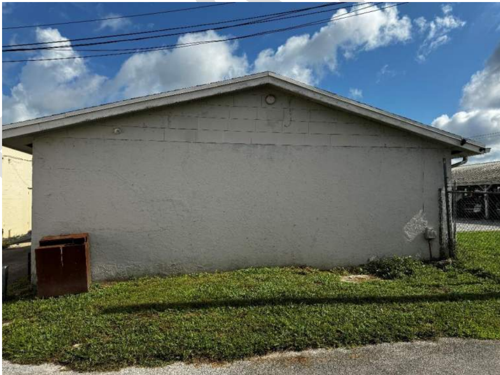
Photo 4 – View of office building south elevation
