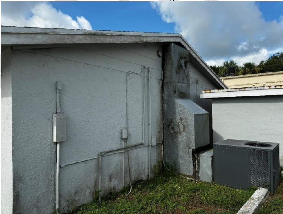
Photo 2 – View of office building north elevation
