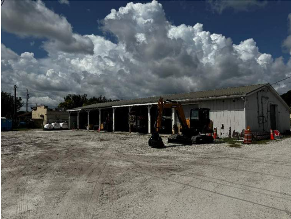
Photo 19 – View of wood shed northeast elevation.
