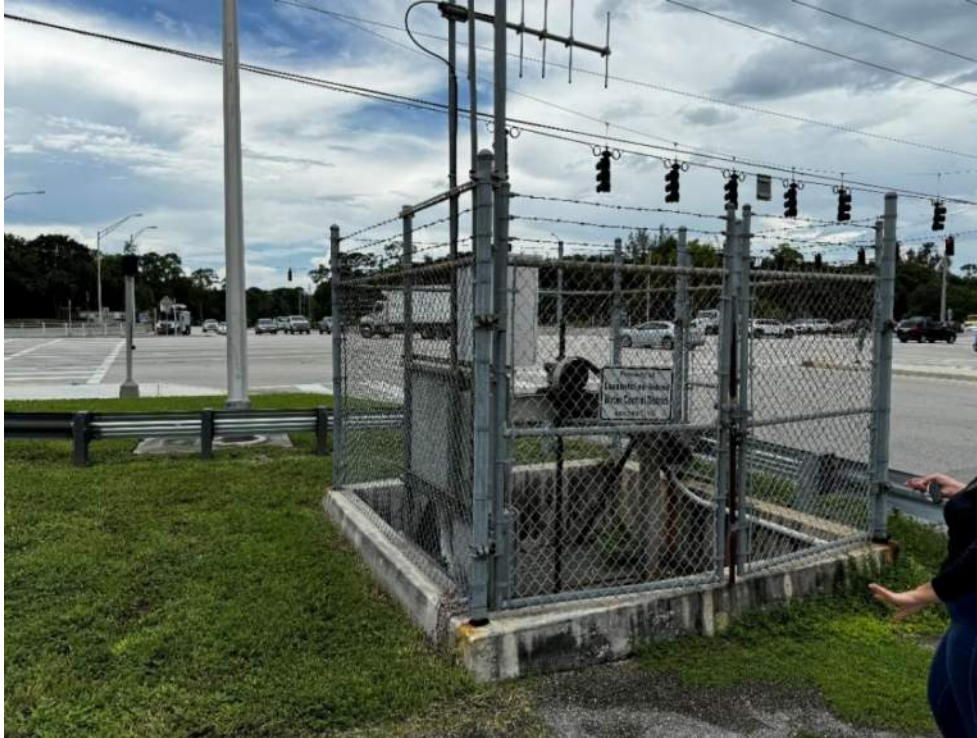
Photo 71 – View of Control Structure C condition.
