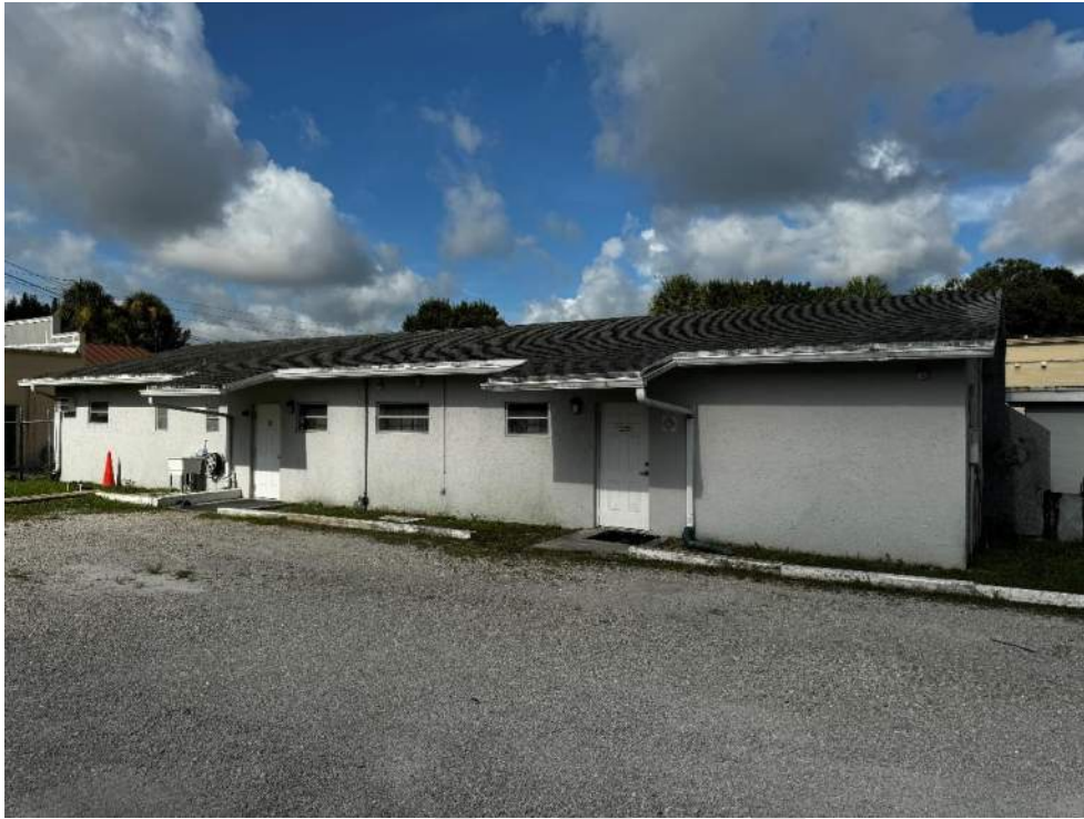
Photo 1 – View of office building east elevation
