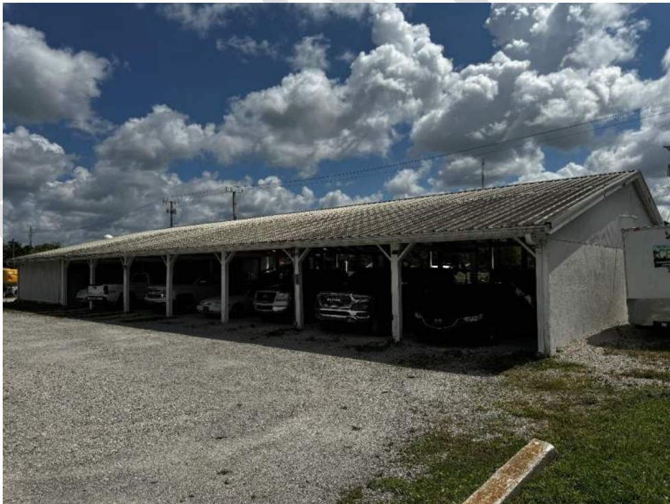
Photo 20 – View of shed southwest elevation.
