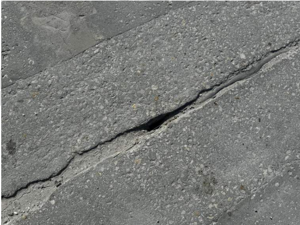
Photo 44 – View of existing expansion joints condition.
