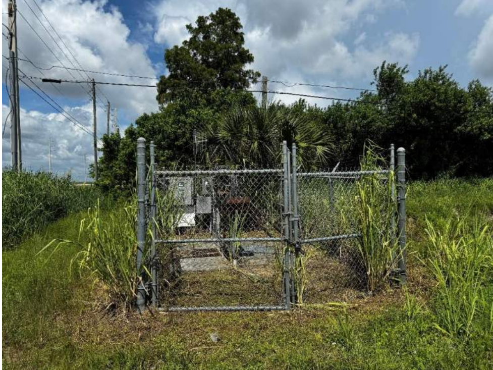
Photo 67 – View of Control Structure A.
