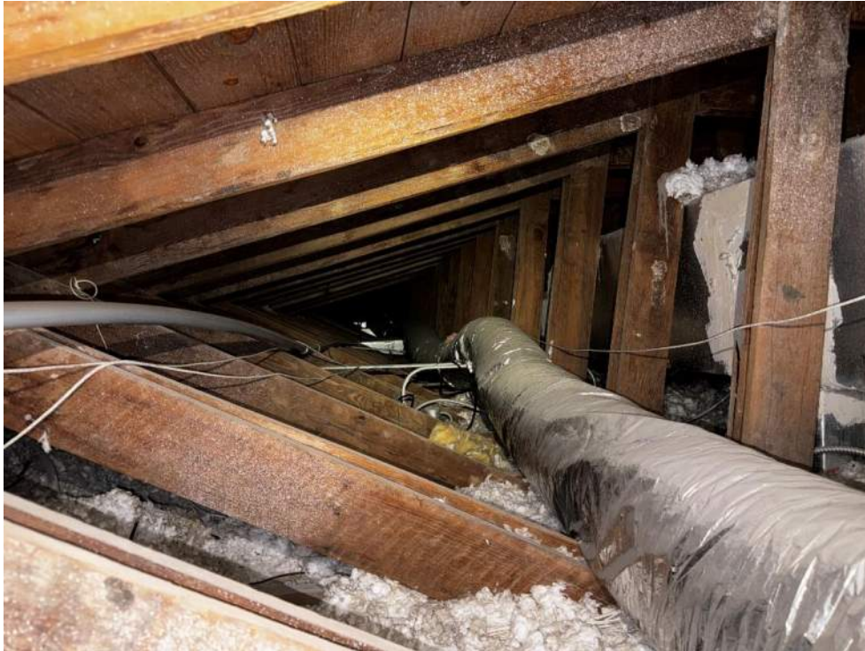
Photo 11 – View of roof wood trusses condition (From north side access hatch).
