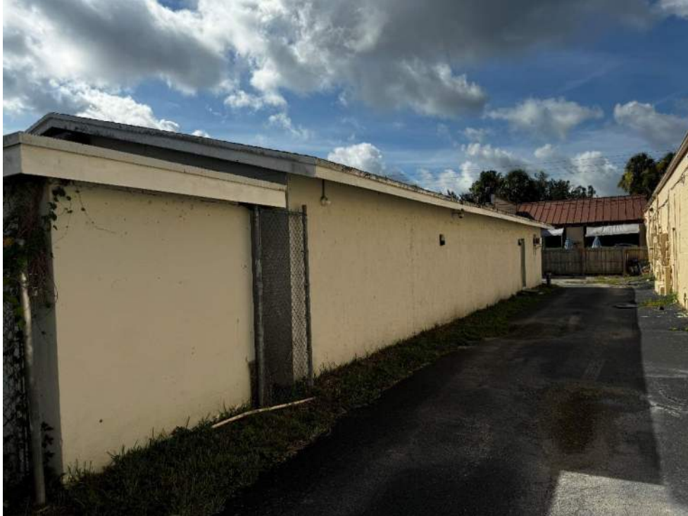
Photo 3 – View of office building west elevation
