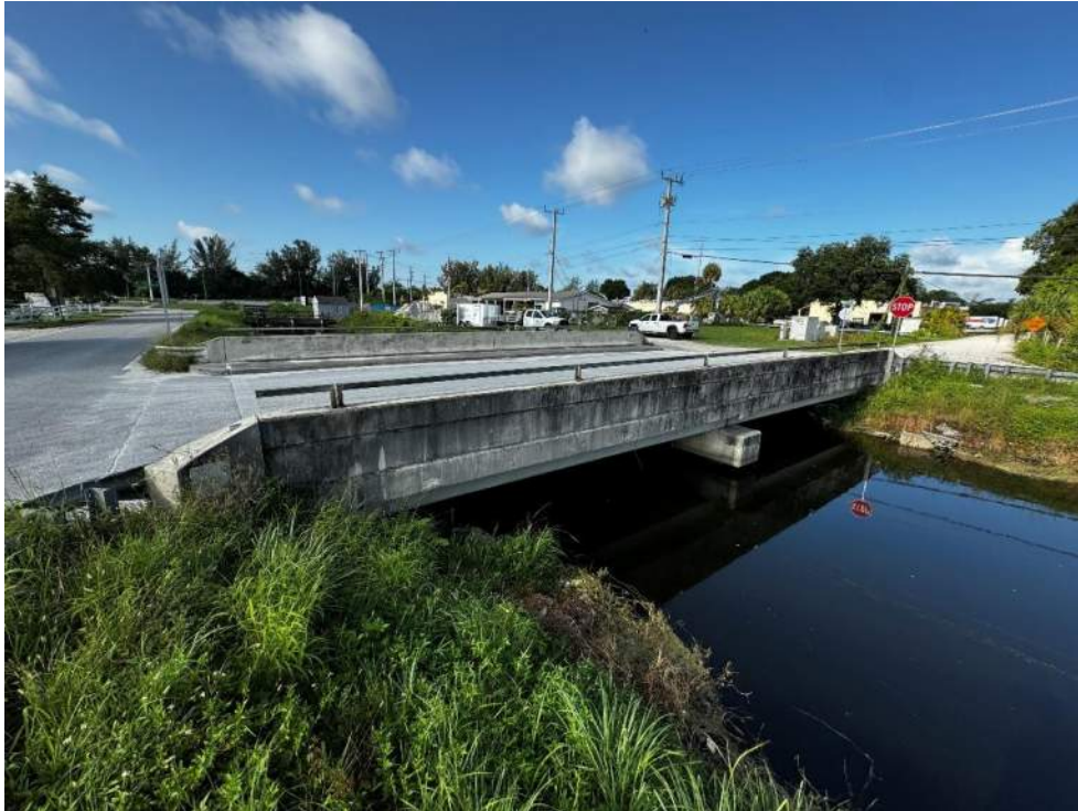
Photo 41 – View of concrete bridge condition.
