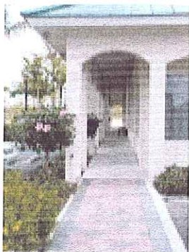
Arches and long colonades
