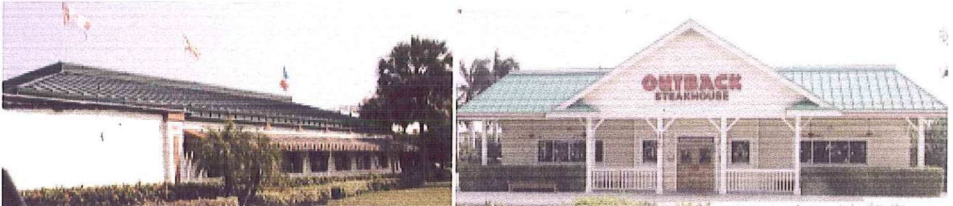
The roofs on these structures are examples of Hip on Deck roof styles.
