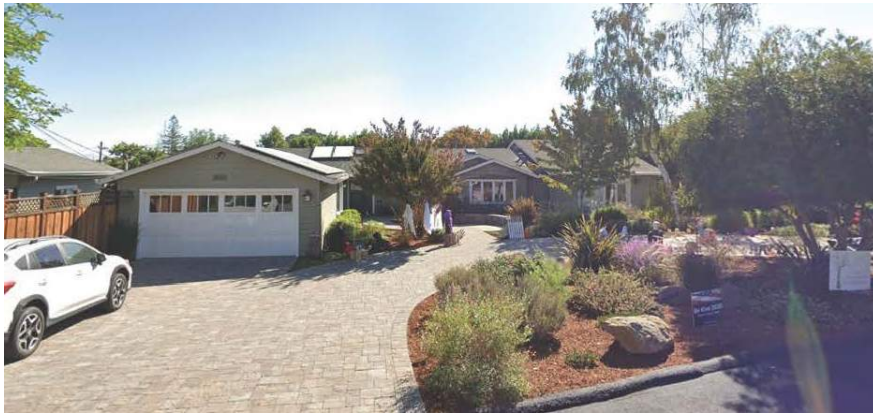
(House next door at 14854 Clara, has gable roof over garage, gabled roof lines, stone used as an accent in middle of façade, and different eave heights.)
