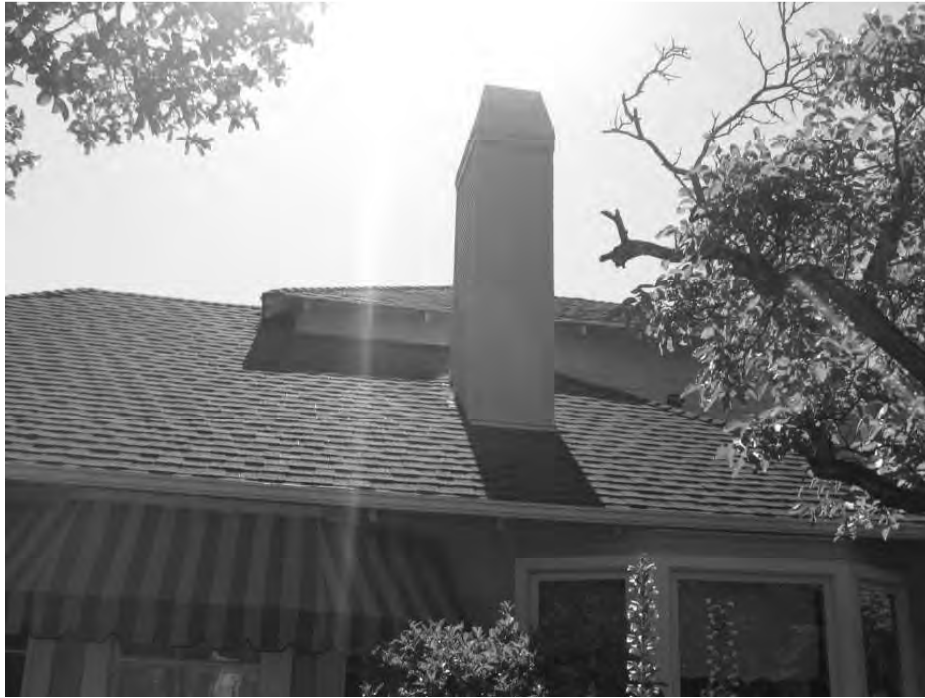
Photo 7: Detail of the (non-original) chimney.
