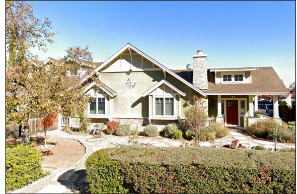
House immediately across Chirco Drive
