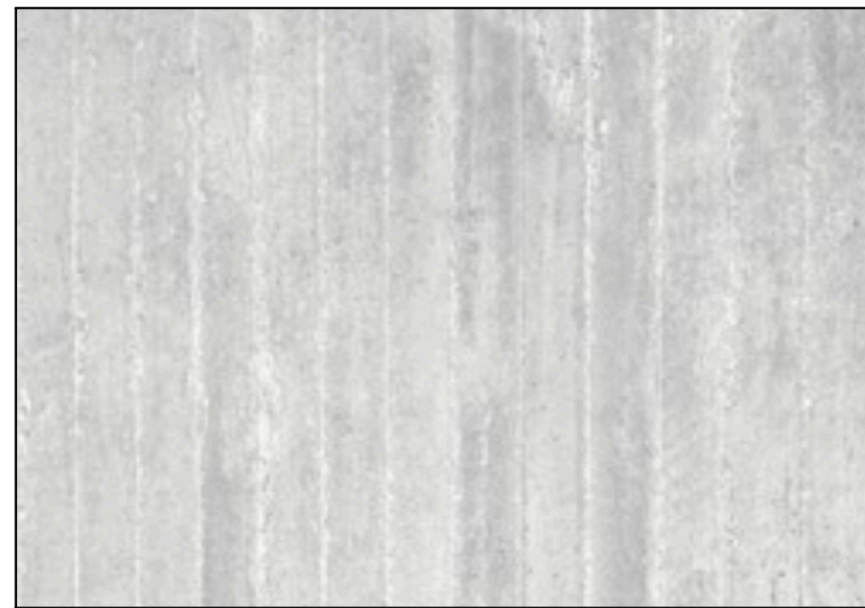
Concrete Accent Wall: Unpainted / Uncovered Light Gray
