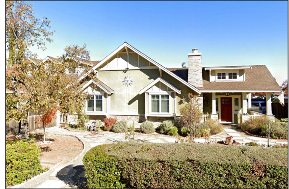
House immediately across Chirco Drive
