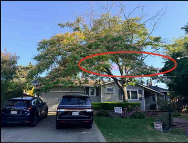
Front View (Covered by a big tree in front of the house)
