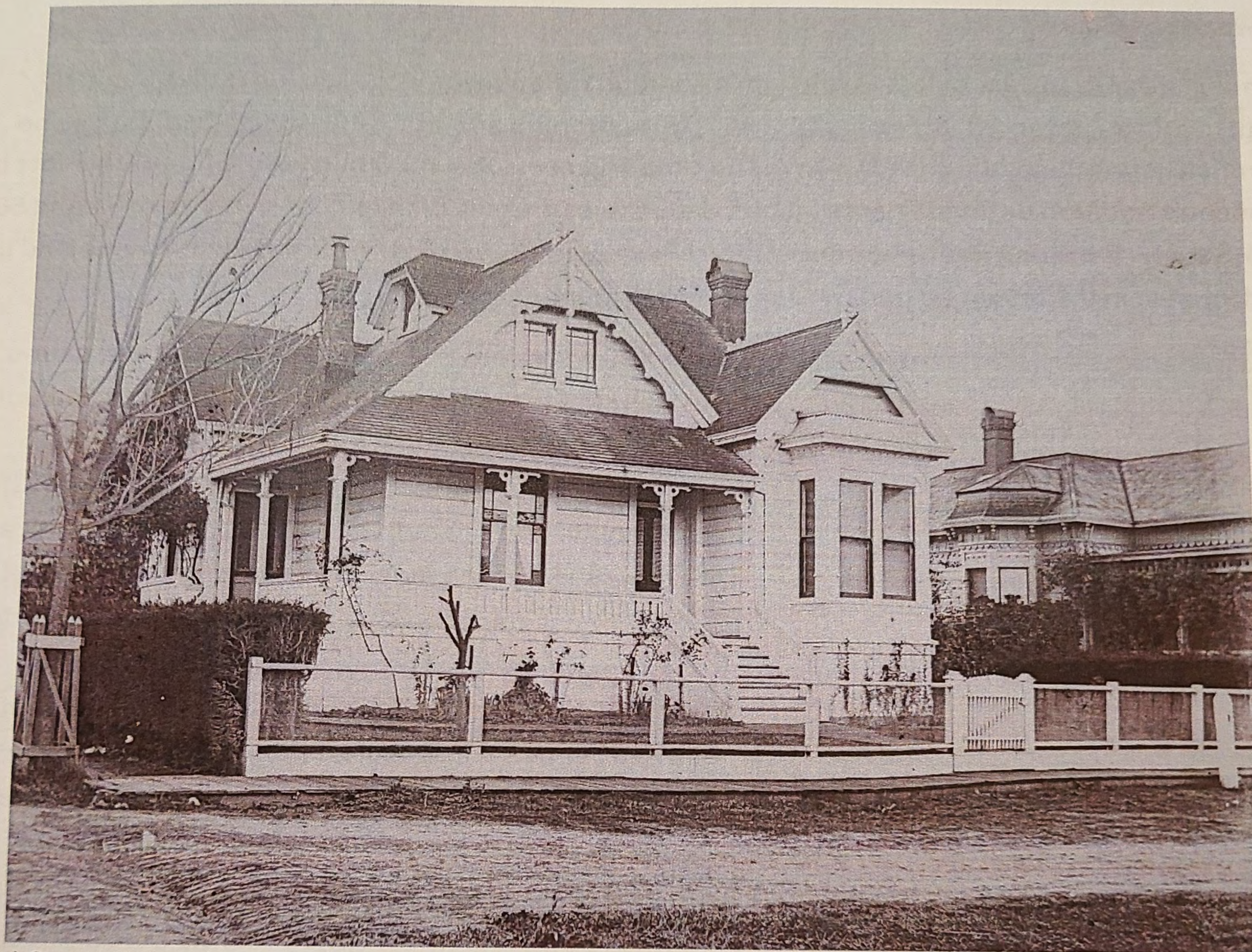
54 Oak Street, photo taken about in 1903, soon after the Snyders moved into the house. The chimney at the right side of the house was the chimney for the parlor fireplace. The chimney came down during the 1906 San Francisco earthquake, and the fireplace was subsequently removed and not replaced. The other chimney would have been for the kitchen stove. The neighboring Victorian house at 50 Oak Street is visible at the right.
