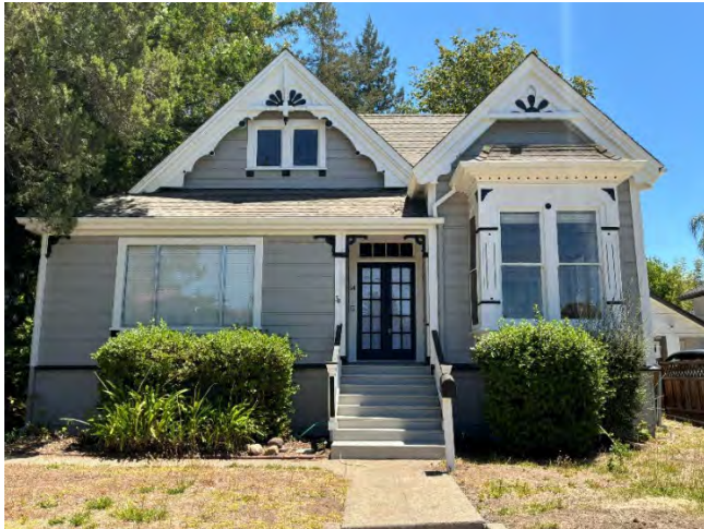
Image B. As Viewed From Whitney Avenue, Present Day
