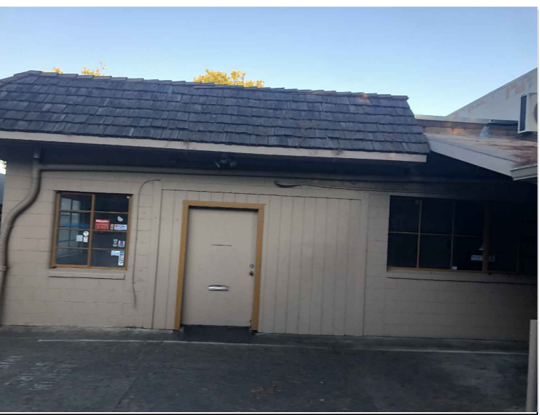
Photo of Rear of Existing Building
