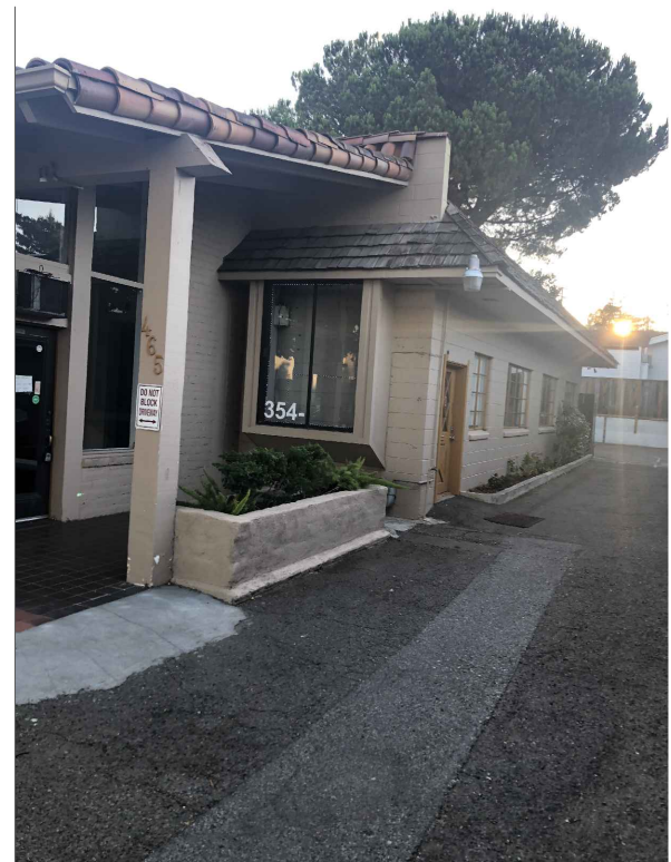
Photo of Side of Existing Building
