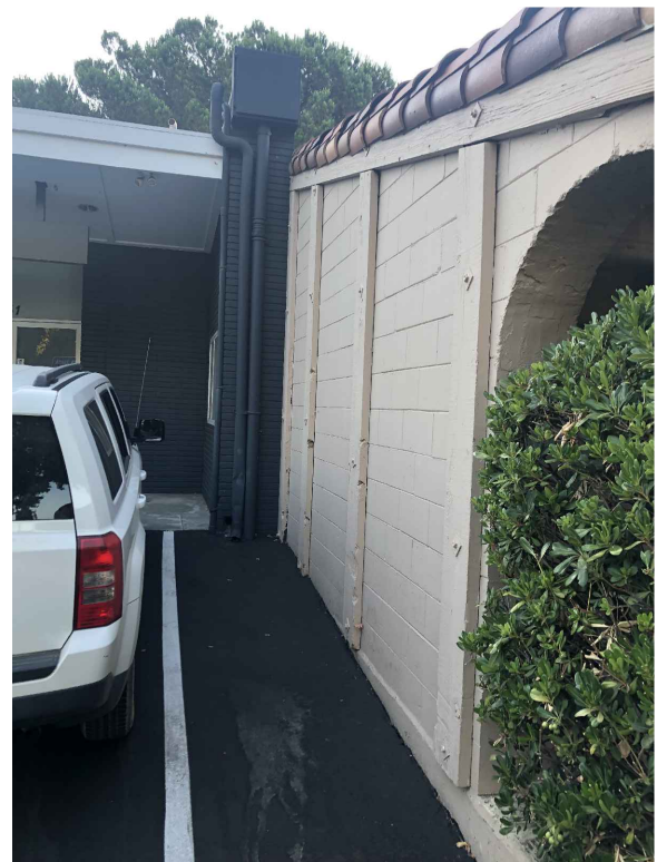
Photo of Side of Existing Building
