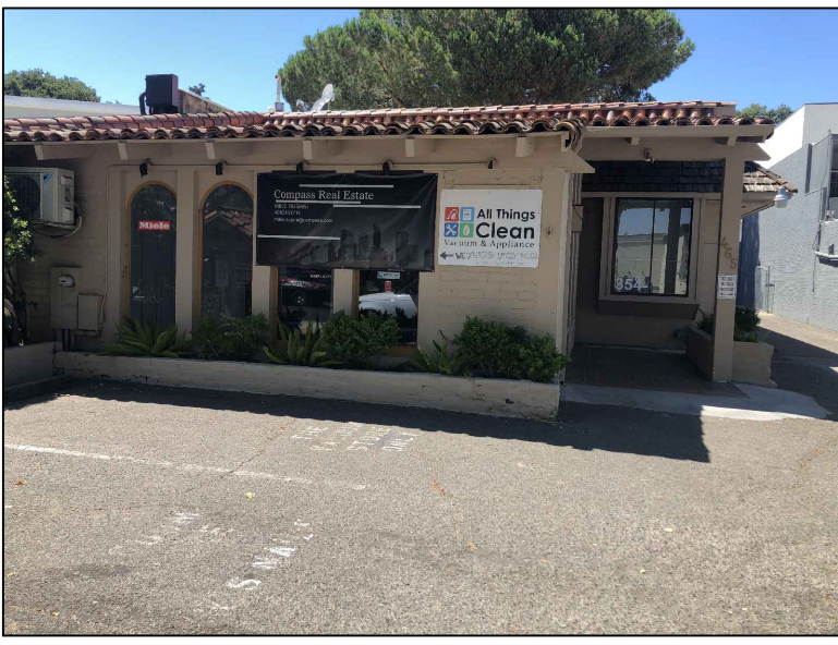
Photo of Front of Existing Building
