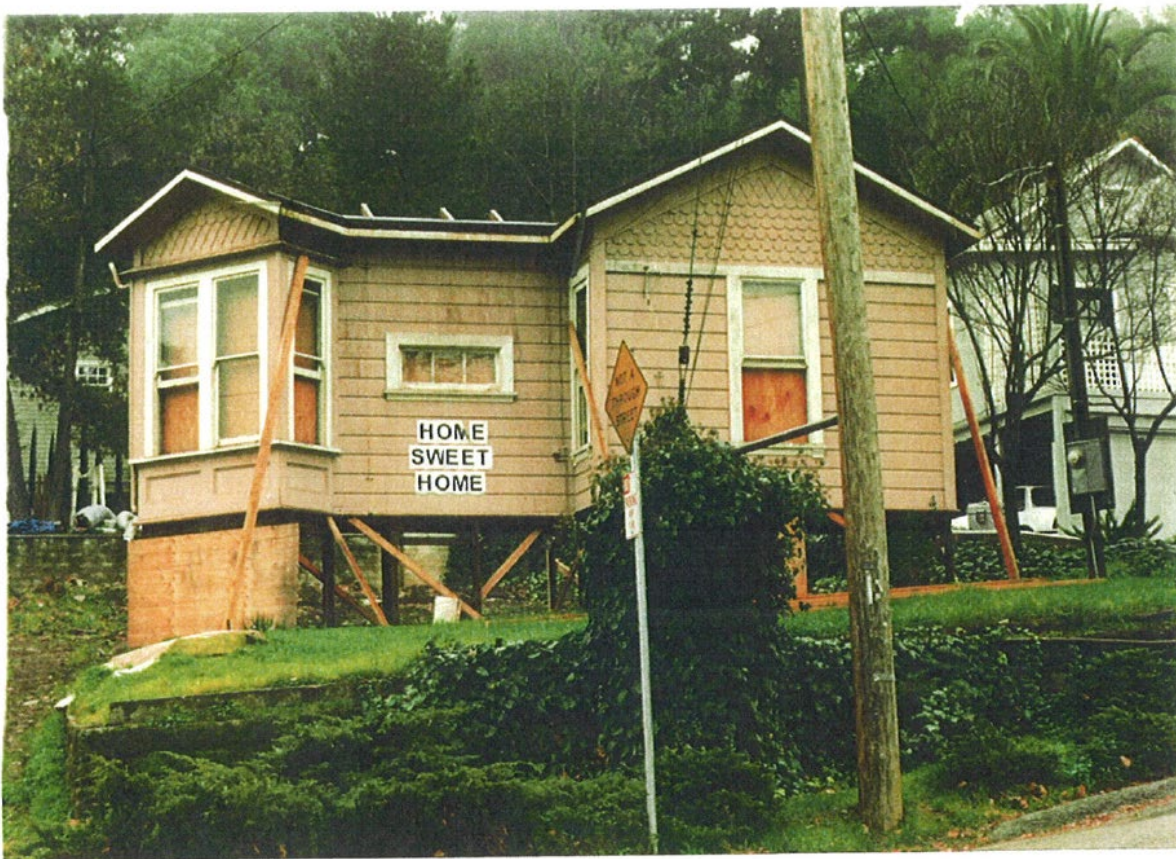
REBUILDING HOUSE AT 93 BROADWAY
