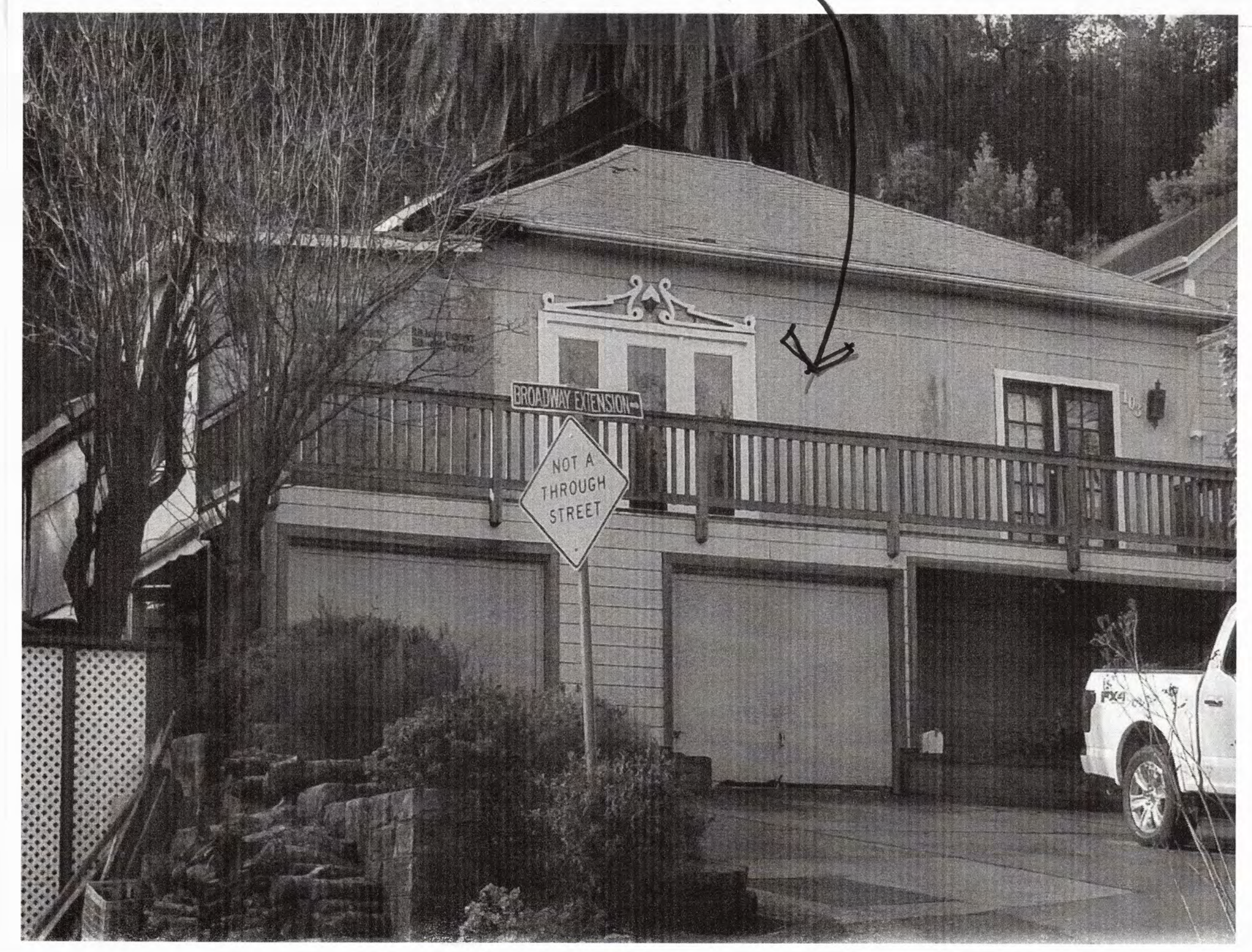
PHOTO OF EXISTING STRUCTURE
