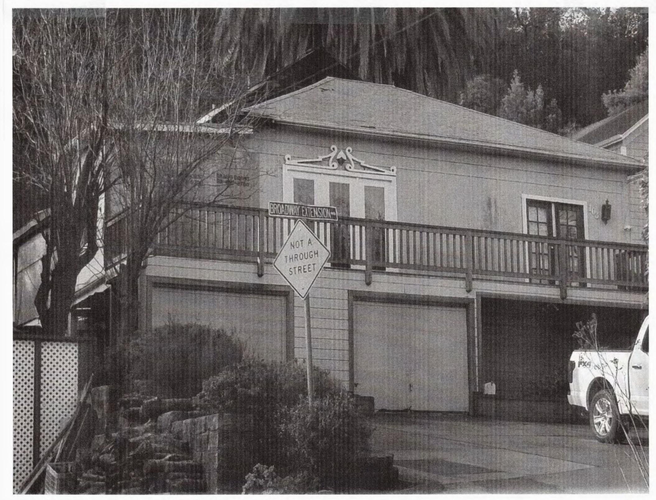
PHOTO of EXISTING STRUCTURE.
