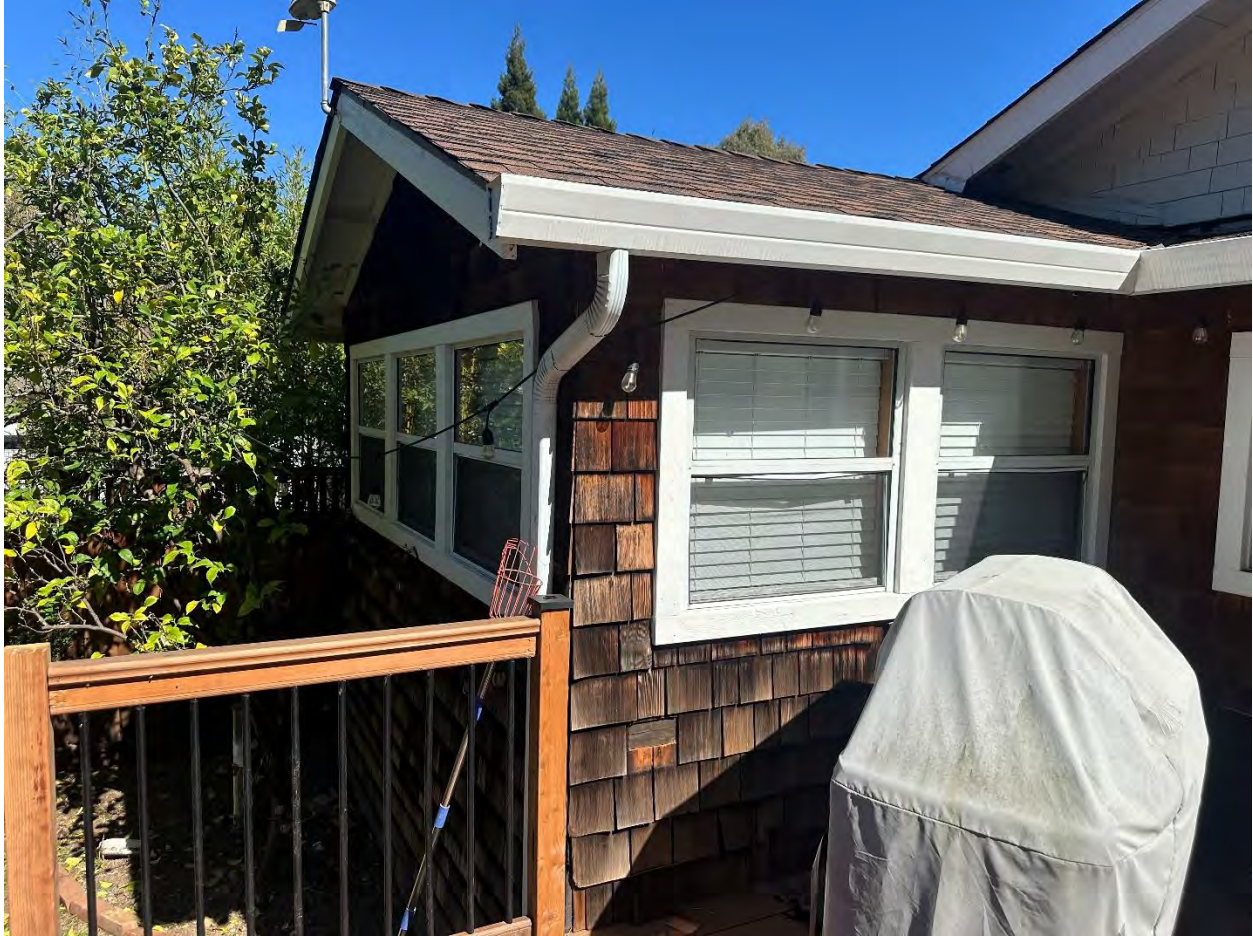
Rear Side post-1956 Constructions
