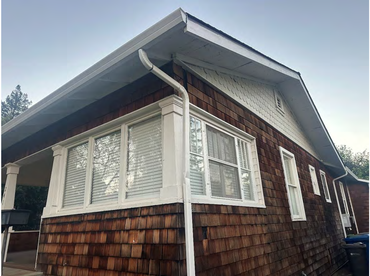
Front Façade + North Side post-1956 Constructions
