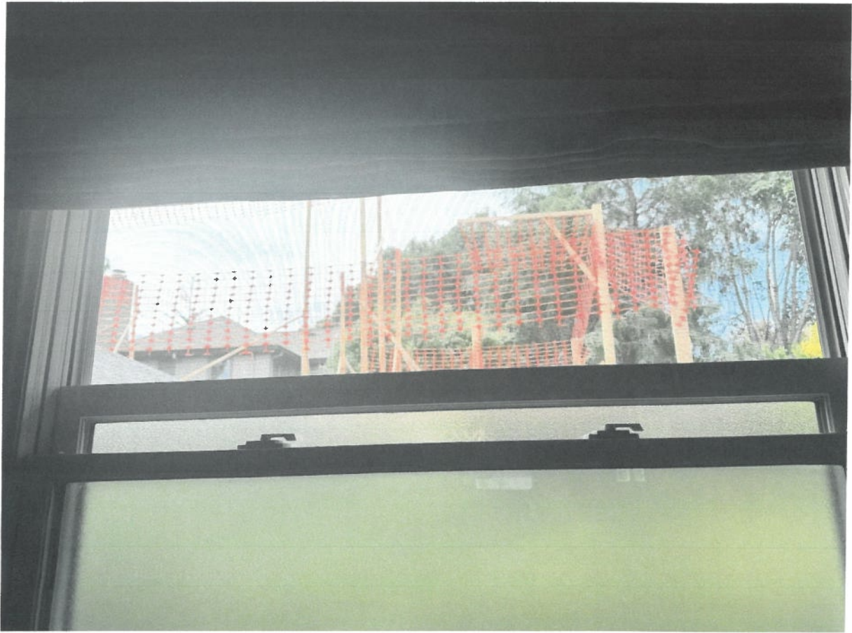
Master Bathroom window over tub
