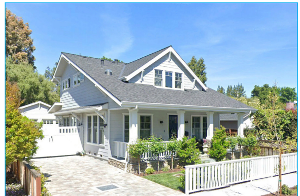
Nearby new house to the right
