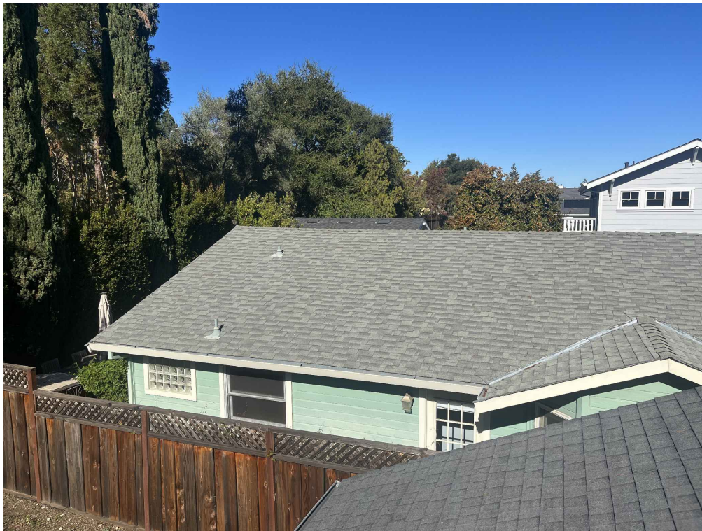
VIEW TOWARDS NORTH:
