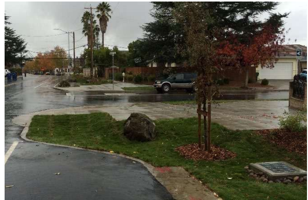
Figure 2-1 Stormwater curb extension, Hacienda Avenue, Campbell (Source: City of Campbell)
