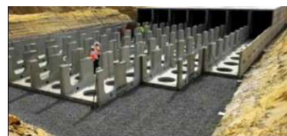
Figure 2-8 Subsurface vault for rainwater harvesting, under construction (Source: Conteches.com)
