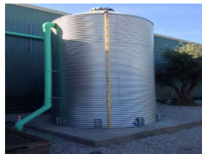
Figure 2-7 Rainwater Harvesting cistern, Environmental Innovation Center, San Jose (Source: City of San José)
