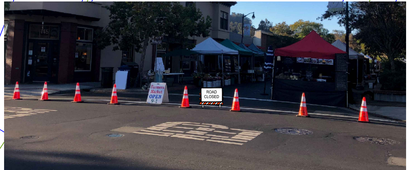
Install 8 traffic cones and one "road closed" sign on A frame
