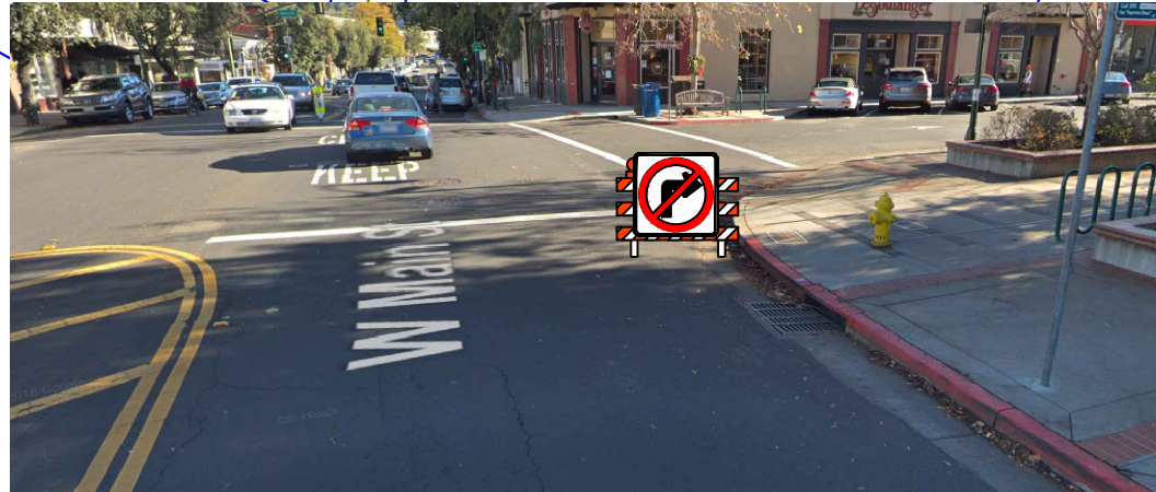
Install a no right-turn sign on A frame
