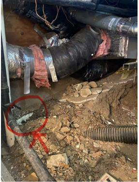
AT FIRST, THE OWNER HAD CONCRETE ADDED TO SEAL AND STABILIZE THE HOUSE. THIS HAS ULTIMATELY FAILED AND NOW THEY APPLY EXPANDABLE SPRAY FOAM TO HELP KEEP OUT RODENTS PERIODICALLY AS THE GROUND BLOW THE FOUNDATION CONTINUES TO SETTLE OVER TIME.
